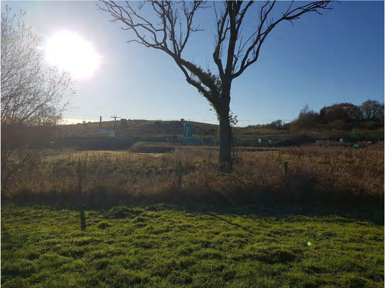
Plate 16 View of Fair Oak Landfill site and gas extraction system
