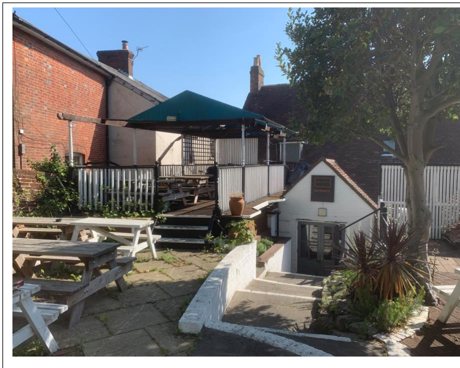
View from street to rear
