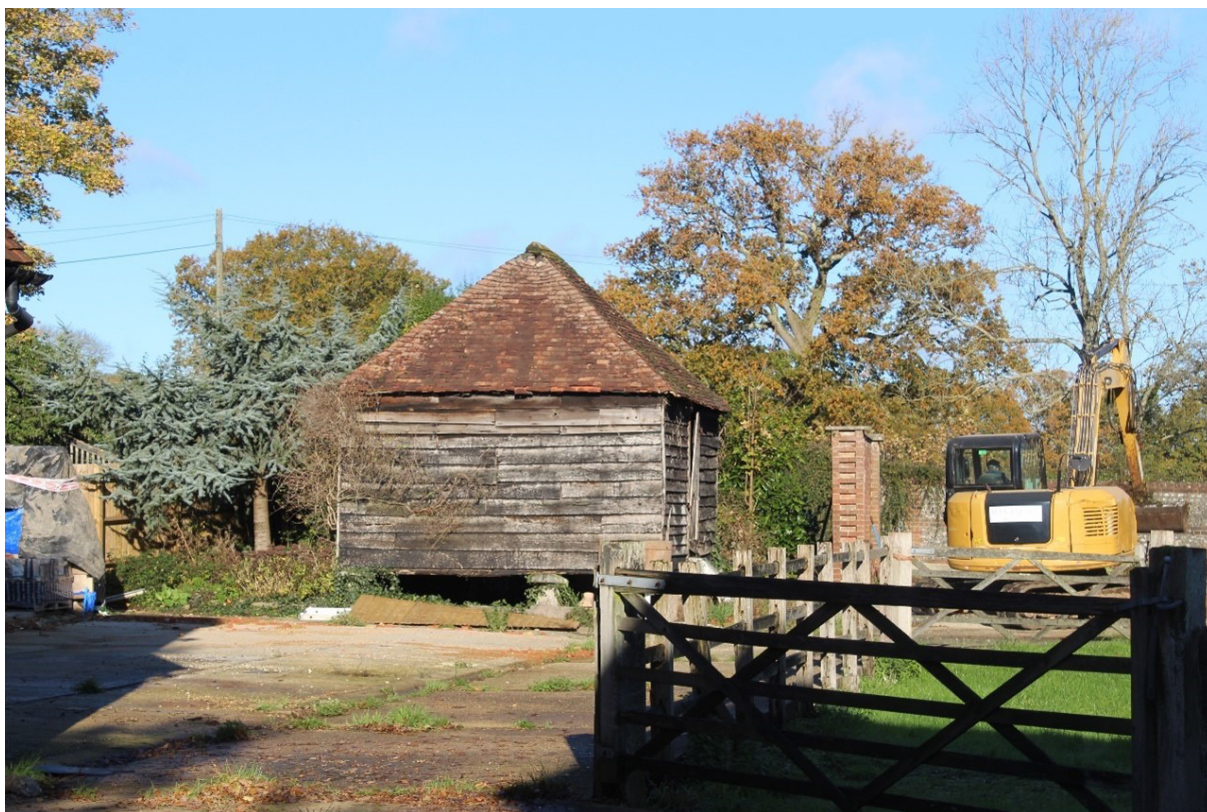
Image EDP A1.4: View of the Grade II listed granary at Mortimers Farm, viewed looking north.
