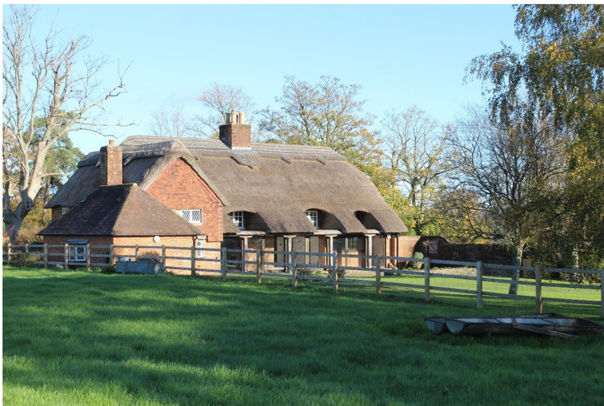
Image EDP A1.2: Mortimers Farmhouse Grade II listed building, looking north from within the fields to the south and illustrating the rear elevation.
