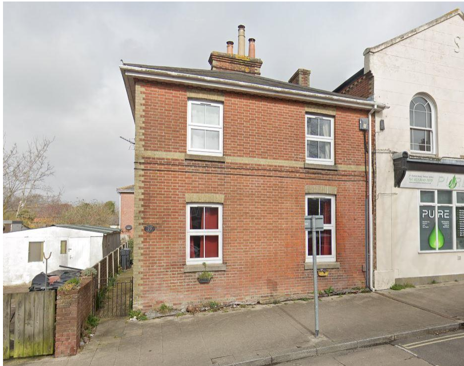
Figure 02 – 19-21 Station Road (Google Streetview extract)
