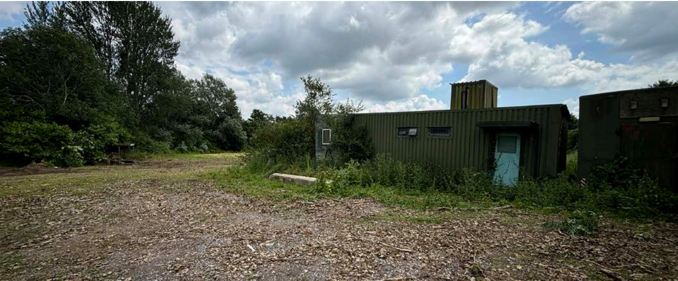
2 Existing Portacabins on Site
