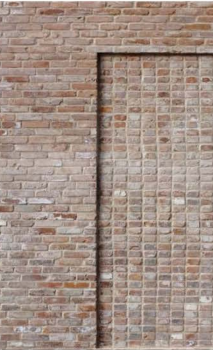
Brick tones and bonding details
