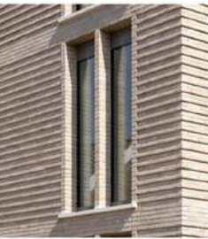
Light Brick with brick sweep detailing to create gradient effect.
