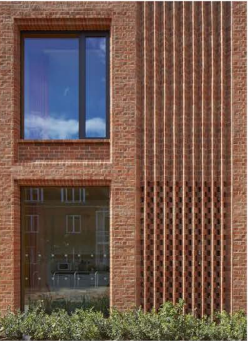
Brick detail, decorative projecting brickwork
