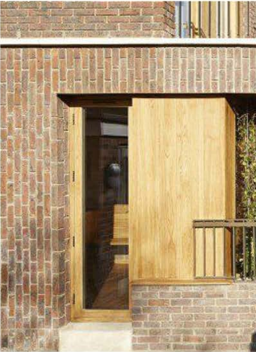
Timber cladding detail
