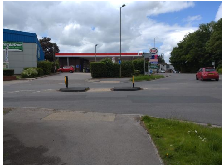
Photograph 4: Dropped kerbs and tactile paving present across roundabout to the north
