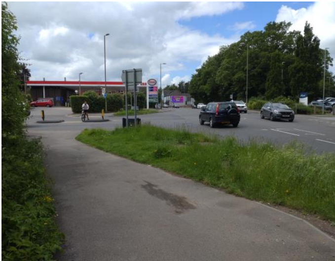
Photograph 3: Existing Footway/Cycleway along Bishopstoke Road
