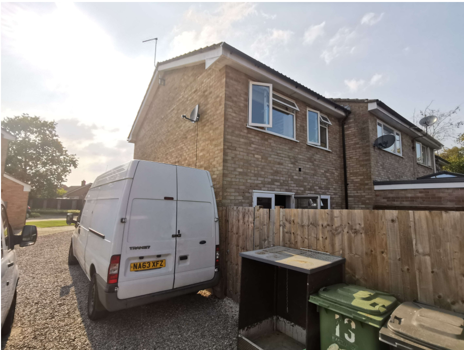
Photograph 03, Existing rear elevation (from East / Driveway)
