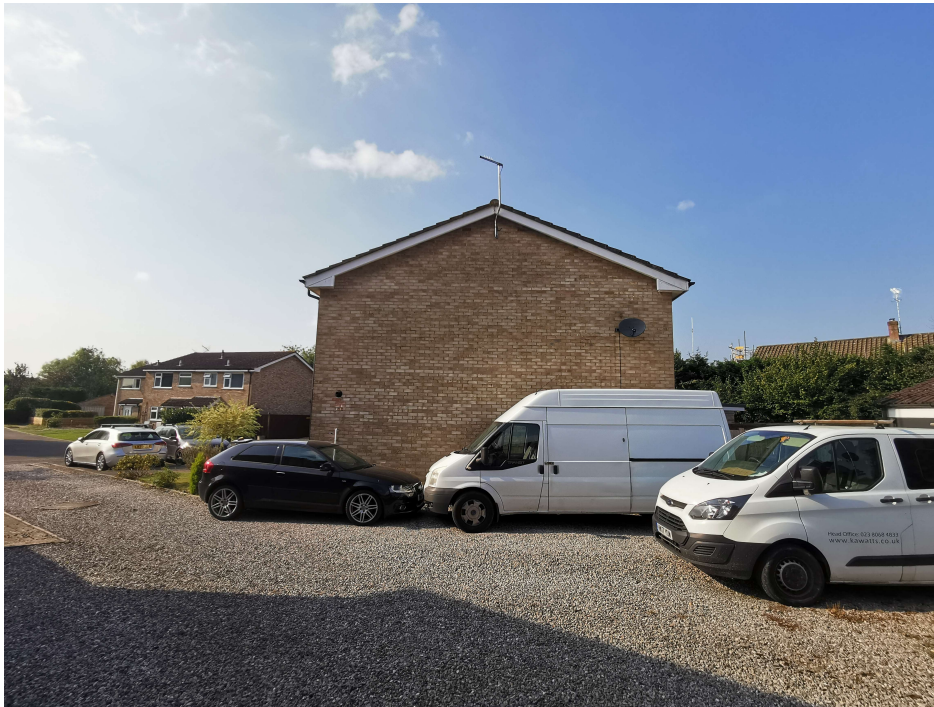
Photograph 02, Existing side elevation (from South / Driveway)
