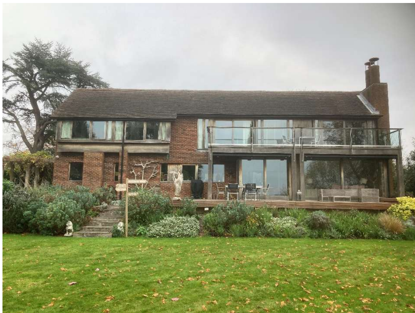
Fig. 5 – Photo taken from the main garden looking towards the south elevation of the house.
