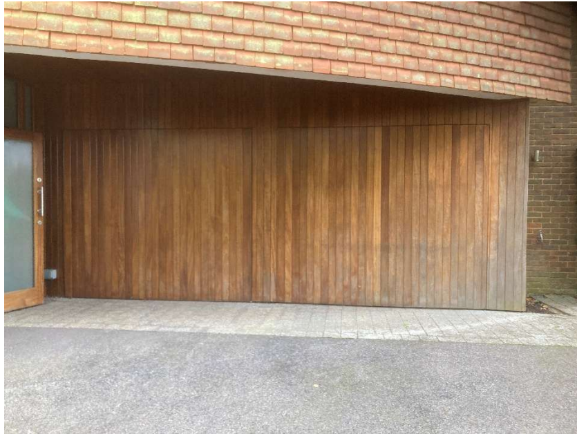
Fig. 4 – Photo taken from the driveway looking towards the timber cladded walls and garage doors on the north elevation.
