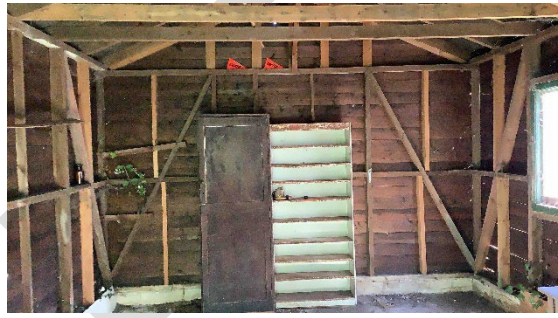
Photograph 12. B2 internal space
