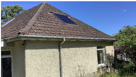
Photograph 3. B1 east aspect
