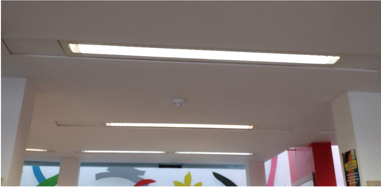
Fig 8: Existing batten and diffuser light fittings.
