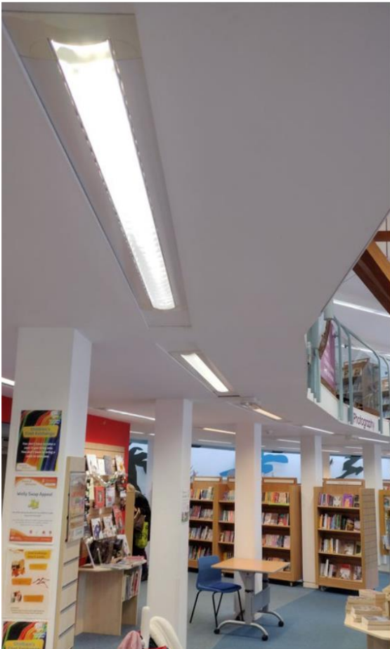
Fig 8: Existing batten and diffuser light fittings.
