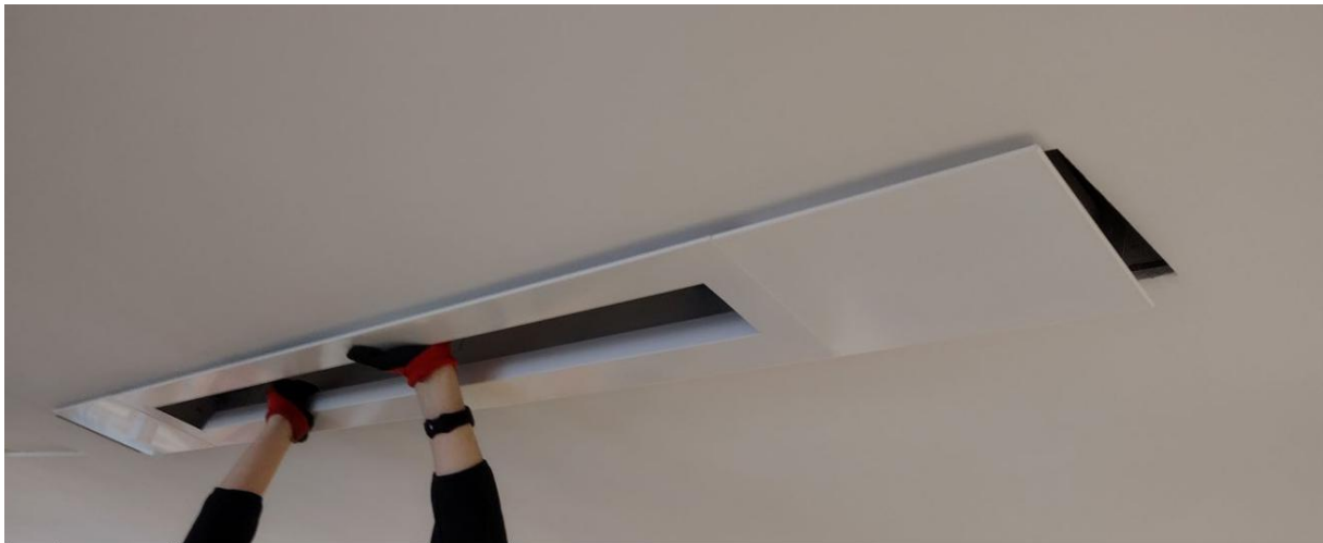
Fig 13: Plasterboard kit trial.
