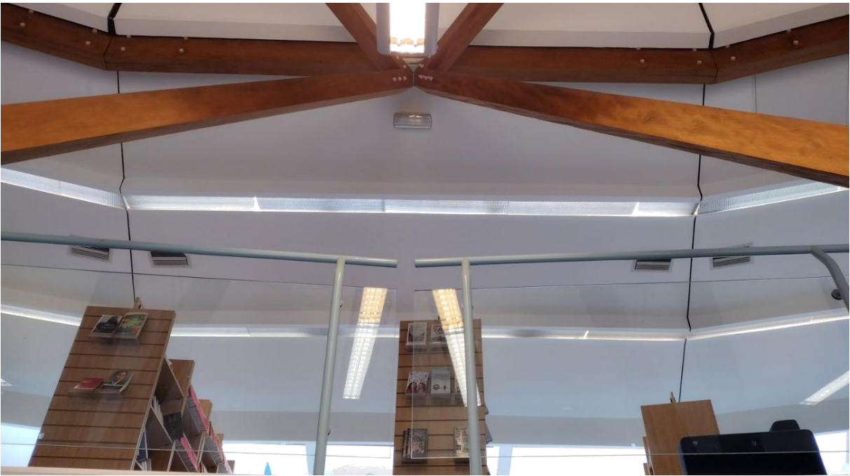
Fig 15: First floor lighting, consisting of batten light fittings fixed into the recess, with an open egg-crate style diffuser.
