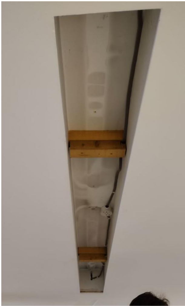
Fig 11 & 12: Existing light removed to show recess; Proposed LED light fitting.
