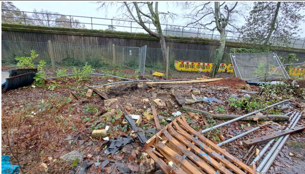
Photograph 2 – AST location following removal. Ground disturbance visible where AST was originally located, no visible staining or odour noted by site team.
