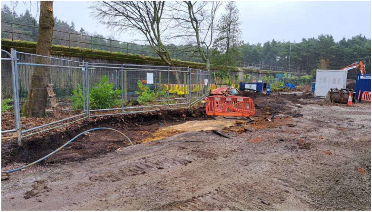
Photograph 3 – AST location following removal and subsequent works
