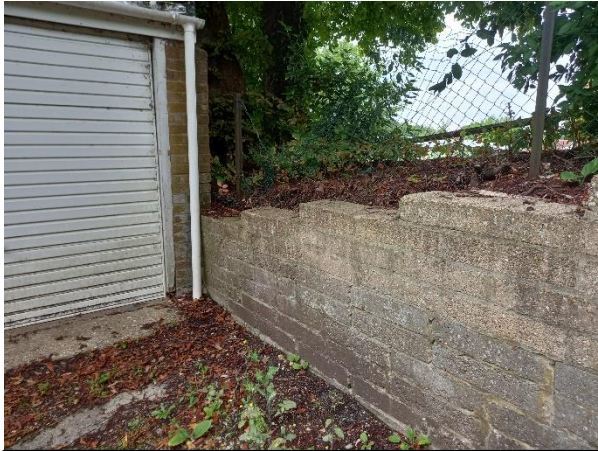
Photo 1: Eastern end of car park where wall adjoins garages. The horse chestnut is in the centre top.
