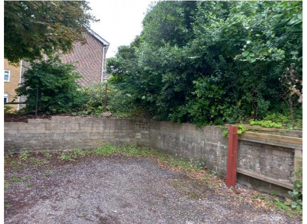
Photo 2: Eastern end of car park where wall turns to form southeastern boundary. Note temporary support.
