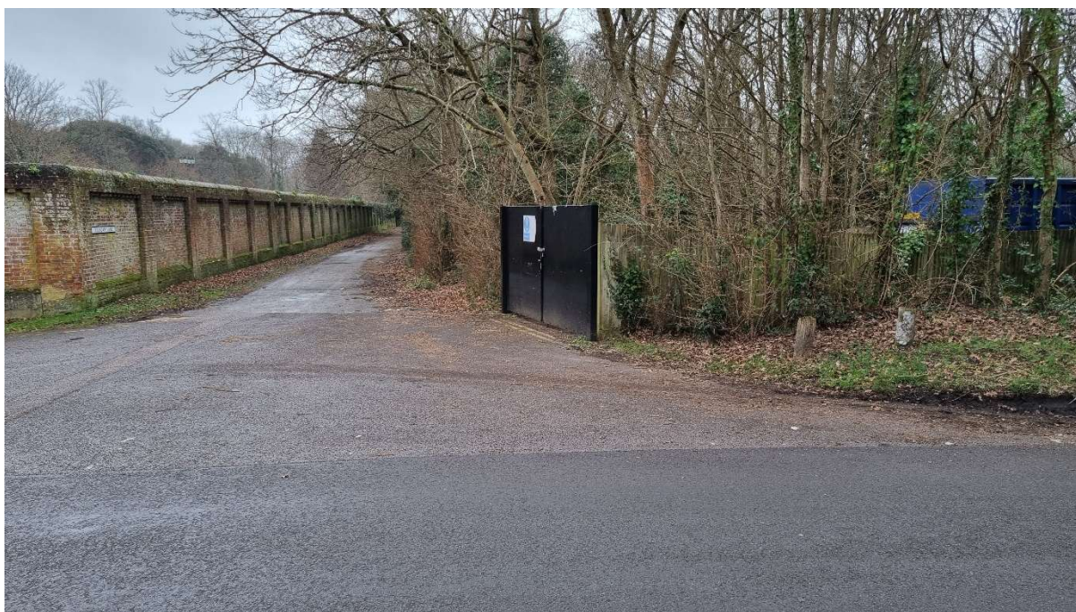
Fig 11: North West corner of Victoria House garden wall. New secure fence & gates to be installed across road.
