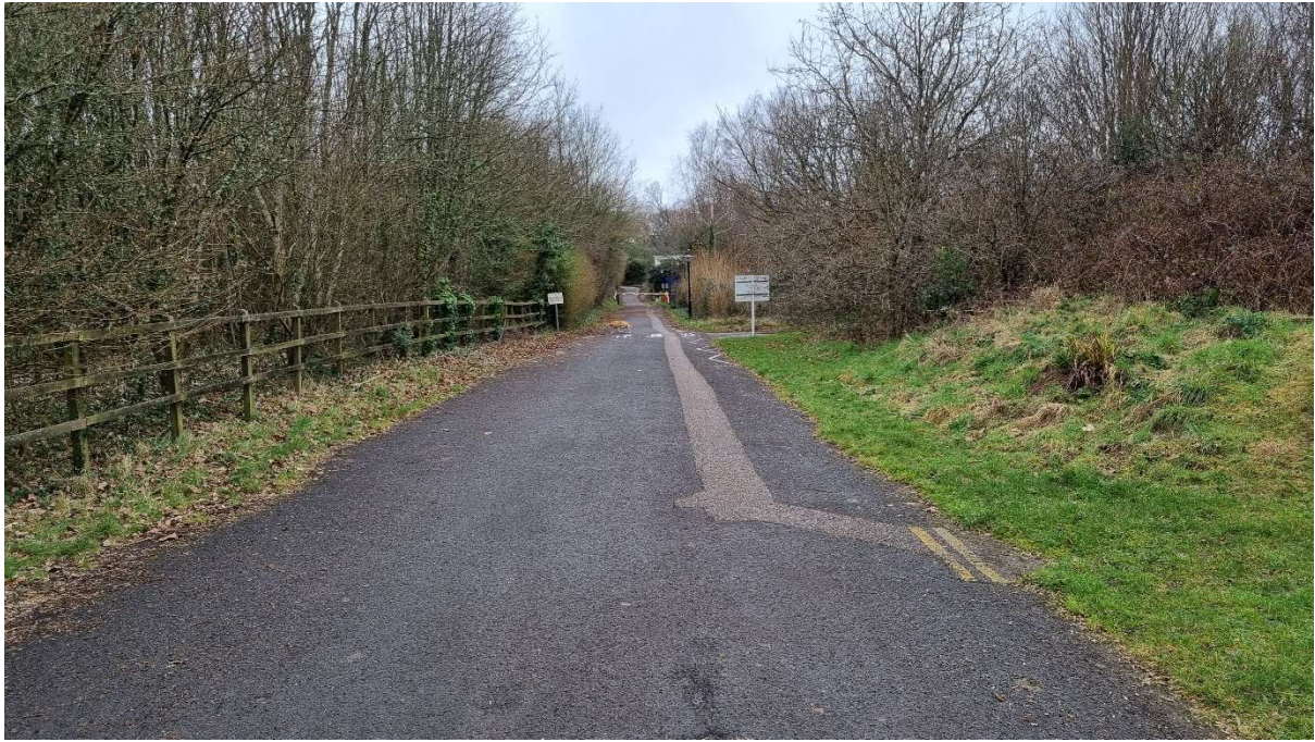
Fig 8: Access road from Hound Road, looking West. New secure gate to be positioned at this point.
