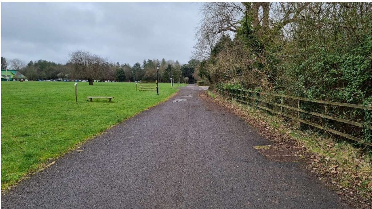
Fig 10: Access road from Hound Road. Secure fence to be positioned to right hand side of road in lieu of timber fence.
