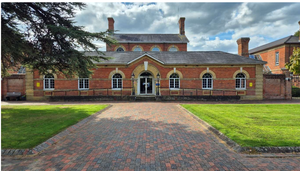
Fig 2: Current view of NE elevation of Victoria House showing main entrance.
