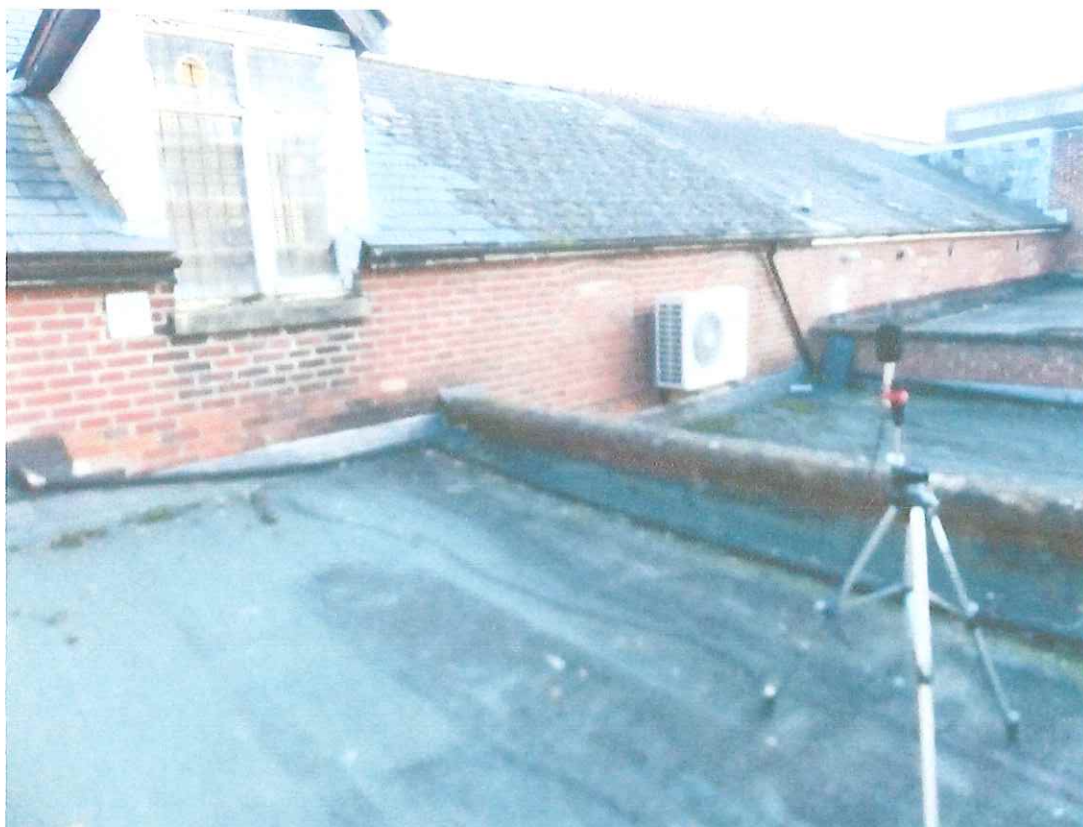
Photo 2 Location 2. On flat roof rear of 11 Market Street premises
