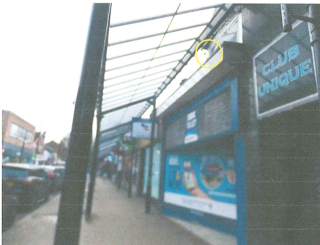
Photo 1 Location 1. 1m ahead of front first floor window
