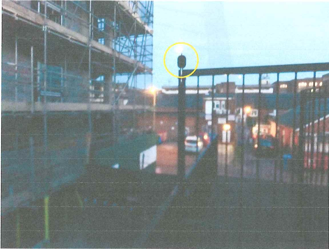
Photo 3 Location 3. On steel staircase at Grayton House
