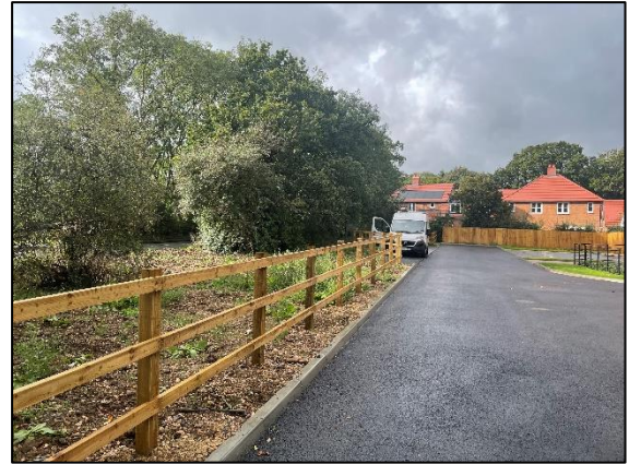
Image 8: Finished surfacing next to T8
