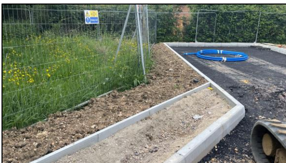
Image 5: Surfacing being finished in southwest corner
