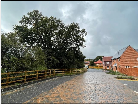
Image 7: Finished surfacing next to T5
