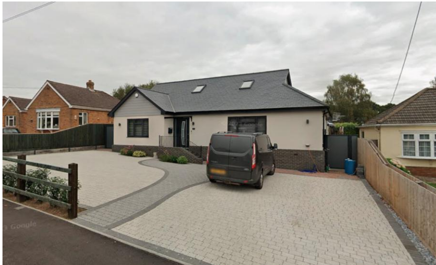
17 Maddoxford Lane – Completed
