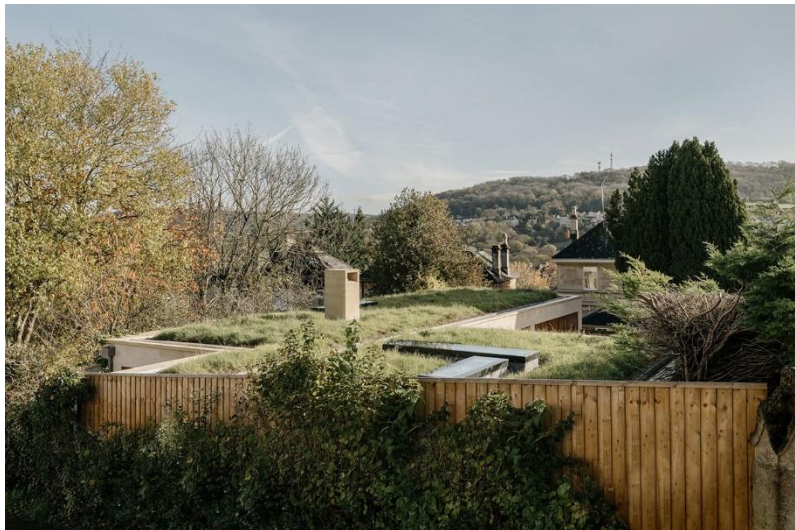
Green Roof Example – Rear Extension
