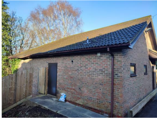
Photograph 8: Southern elevation of the building.
