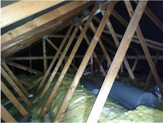
Photograph 13: View of the roof void.
