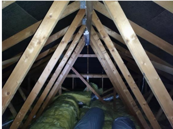
Photograph 12: View of the roof void.
