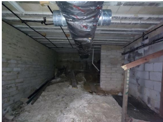
Photograph 18: View of the southern side of the basement.
