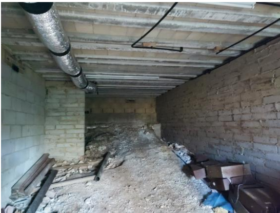
Photograph 17: View of the northern half of the basement
