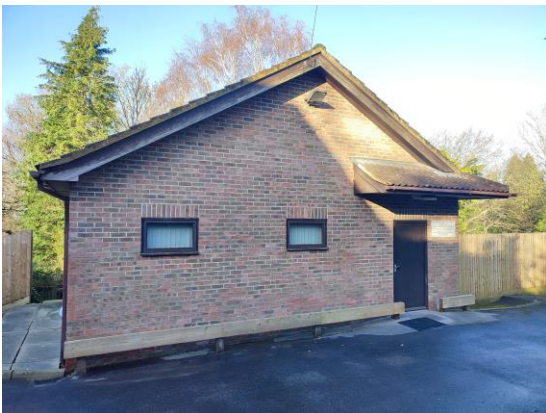
Photograph 5: Eastern elevation of the building.
