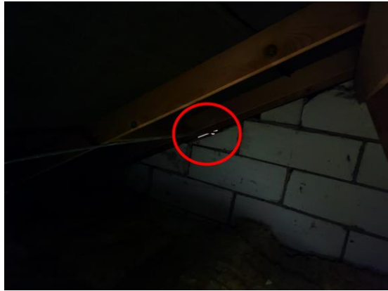
Photograph 16: Light can be seen entering the roof void through a gap in the gable end on the eastern side of the roof void.
