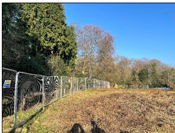
Image 5: Tree protection barriers along western boundary adjacent to trees H10—T17
