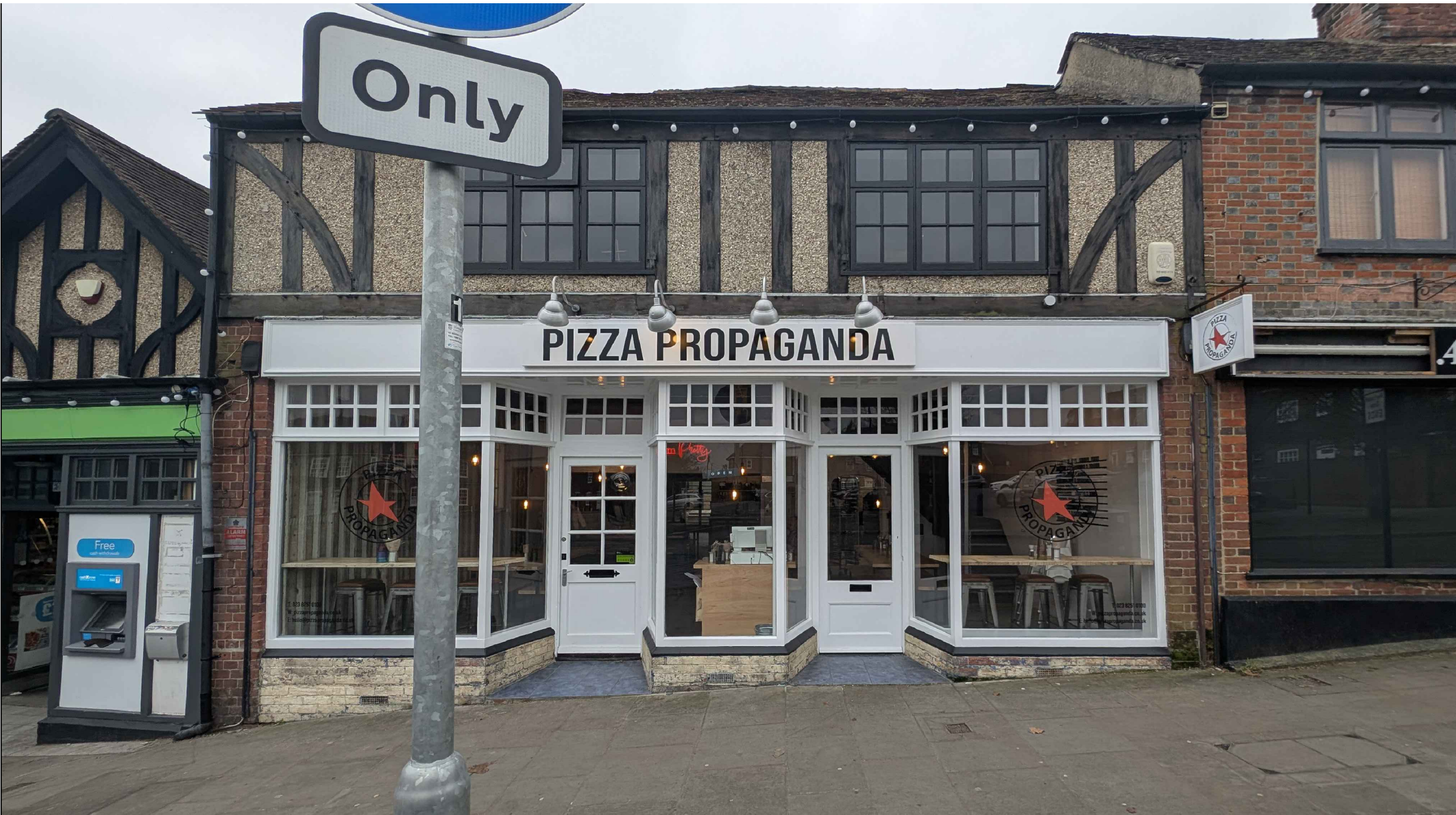
CURRENT SIGNAGE ON EXISTING ILLUMINATED SHOP FRONT SIGN BOARD
