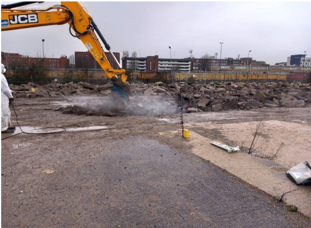
Plate 12: Site Visit 22/12/22 – Dust suppression during breakout with Air Monitoring
