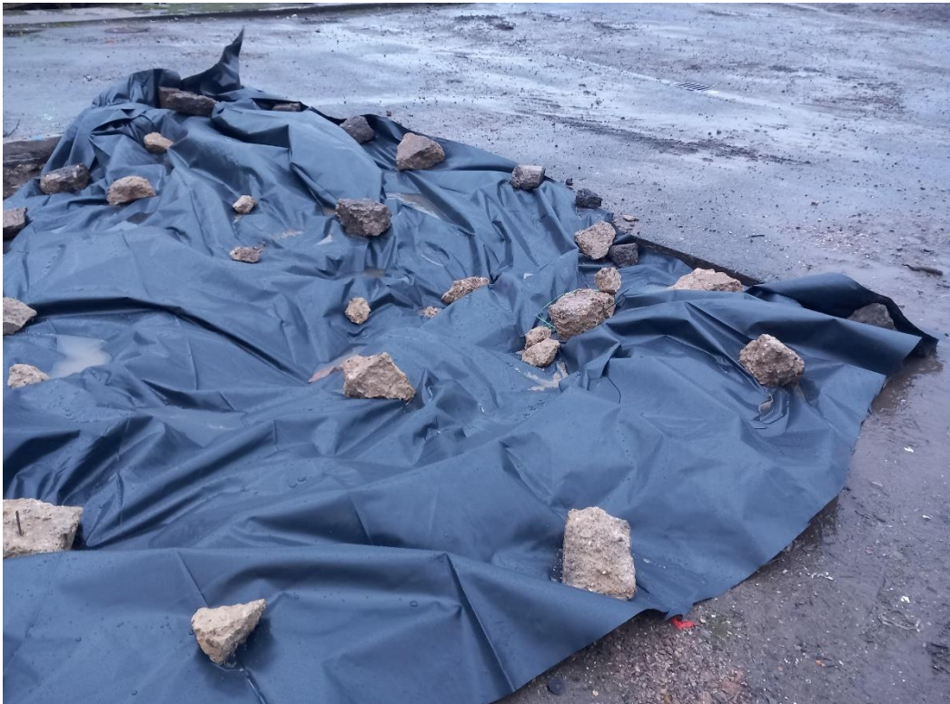
Plate 11: Site Visit 19/12/22 – Covered suspected asbestos
