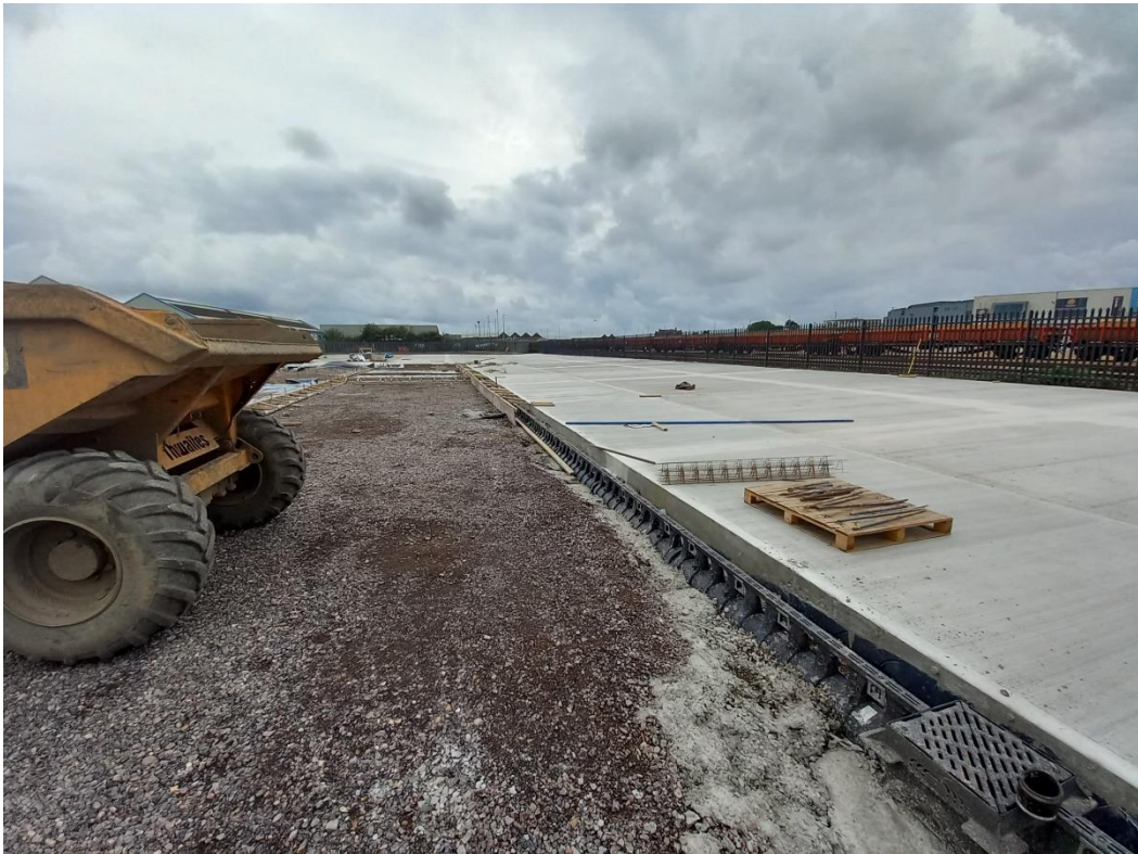
Plate 34: Site Visit 04/07/23 – Installation of concrete surfacing.
