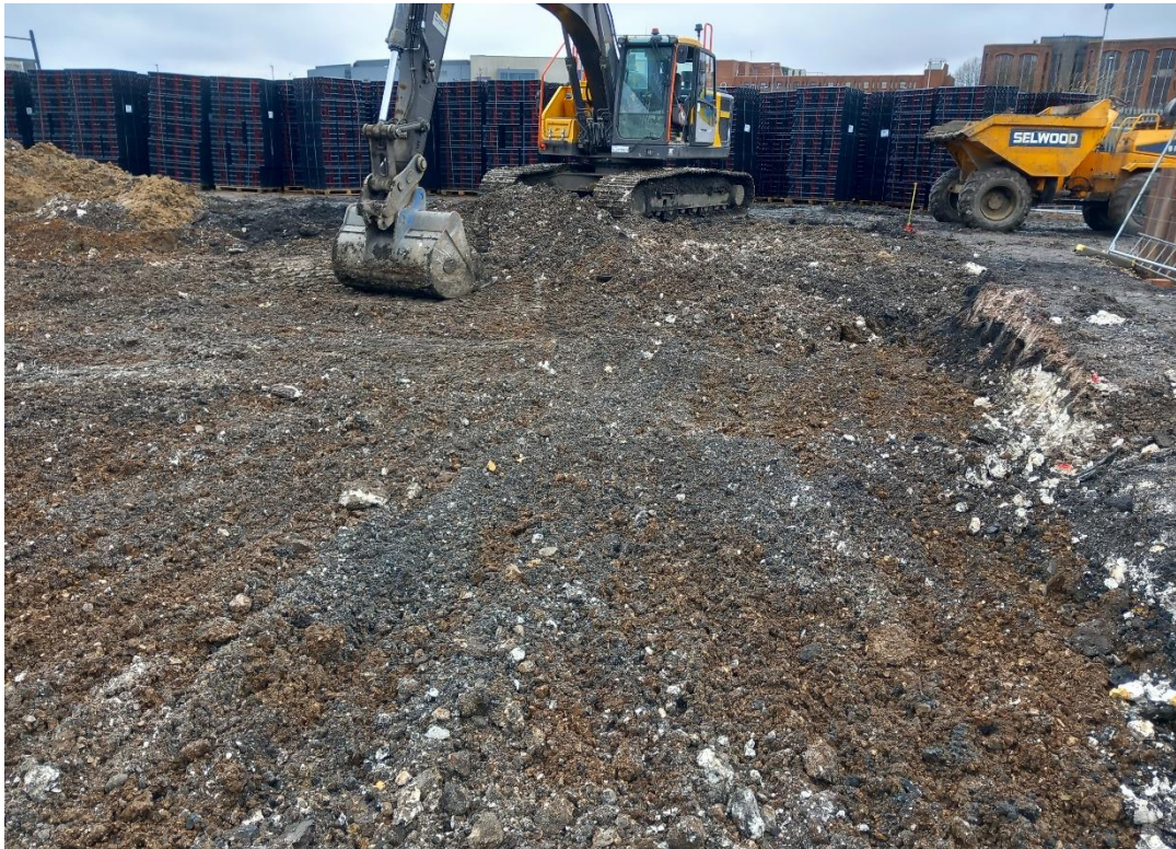
Plate 31: Site Visit 21/03/23 –Continued excavation to formation level
