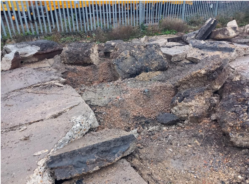
Plate 9: Site Visit 19/12/22 – Surface hardstanding breakout in the west of the site
