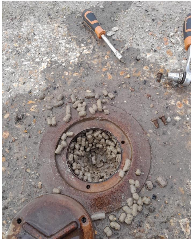
Plate 5: Site Visit 06/12/22 – WS06 confirmation of decommissioning
