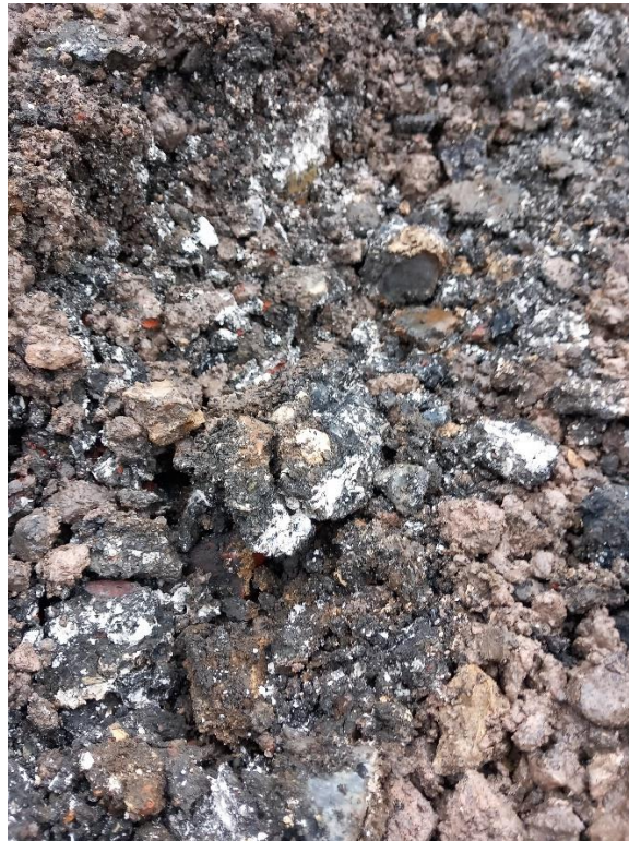
Plate 8: Site Visit 19/12/22 – Suspected ACM (lagging) observed in excavation of the vicinity of WS05
