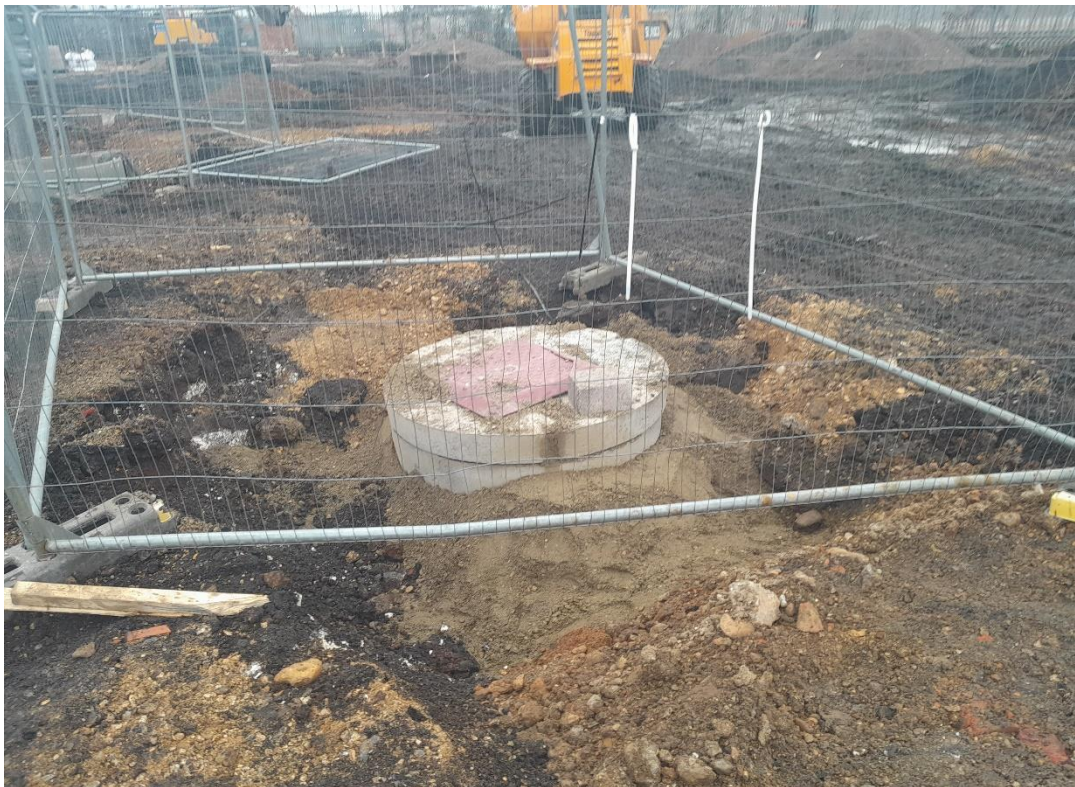
Plate 24: Site Visit 24/01/23 – Manhole chamber installed
