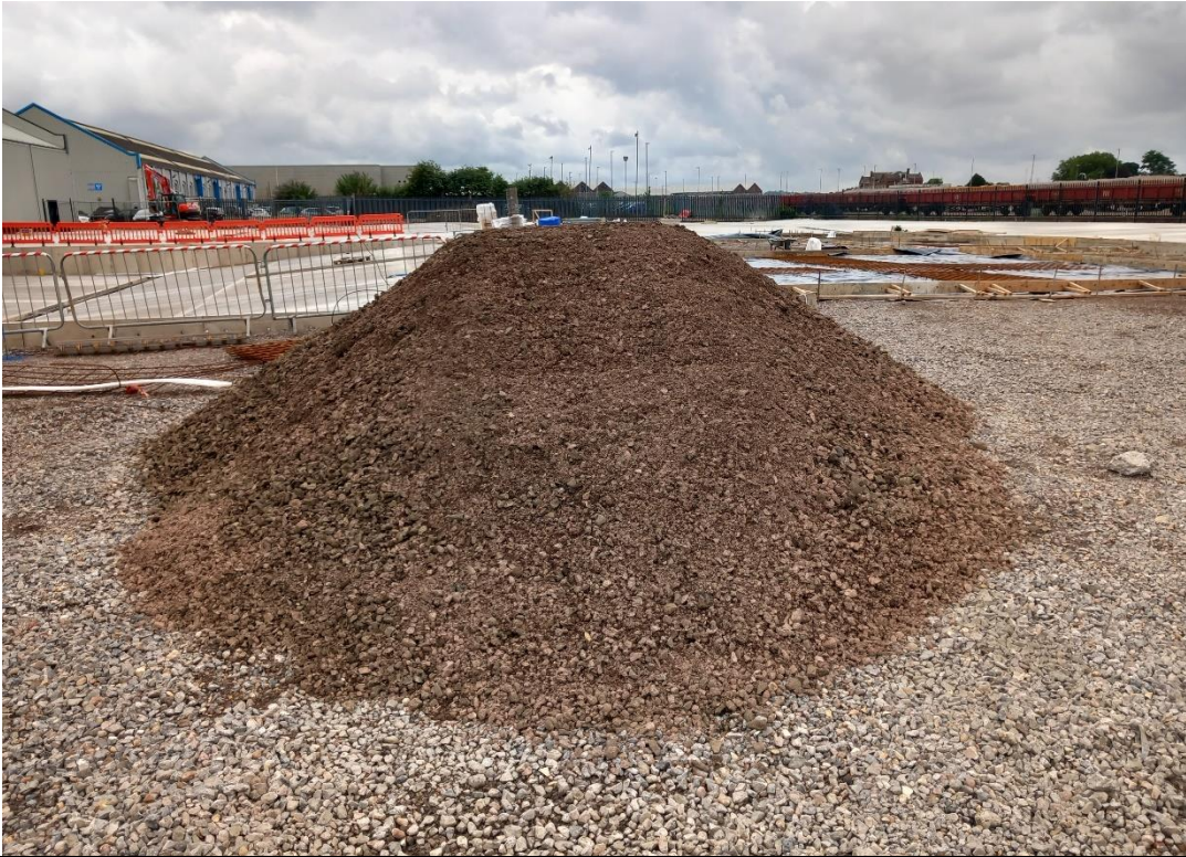
Plate 33: Site Visit 04/07/23 –Imported material for subbase
