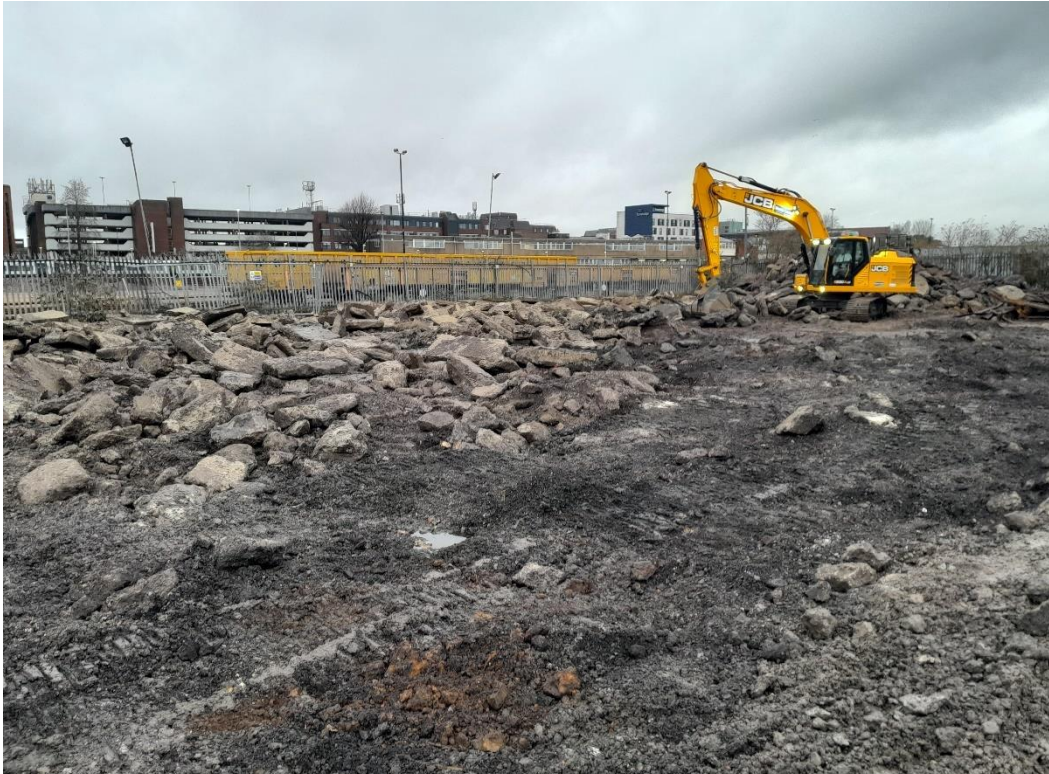
Plate 19: Site Visit 04/01/23 – Continued concrete breakout and soil inspection along western boundary
