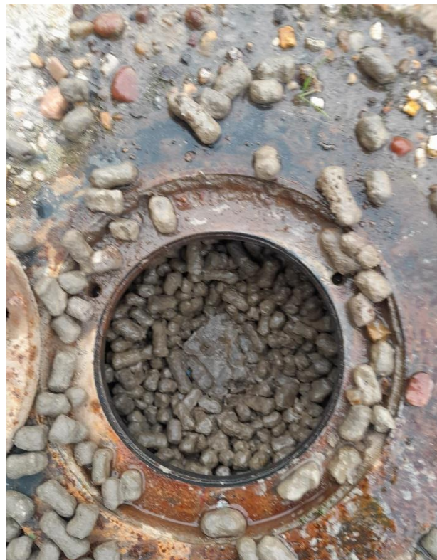
Plate 6: Site Visit 06/12/22 – WS07 confirmation of decommissioning
