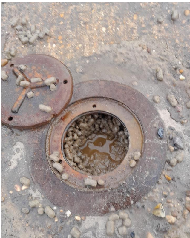
Plate 4: Site Visit 06/12/2022 – WS05 confirmation of decommissioning
