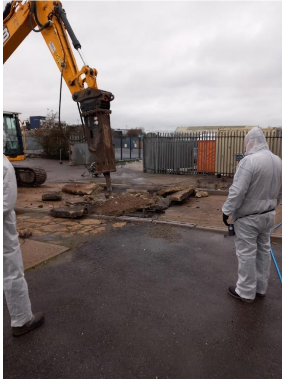
Plate 7: Site Visit 19/12/22 – Commencement of concrete breakout near to WS05
