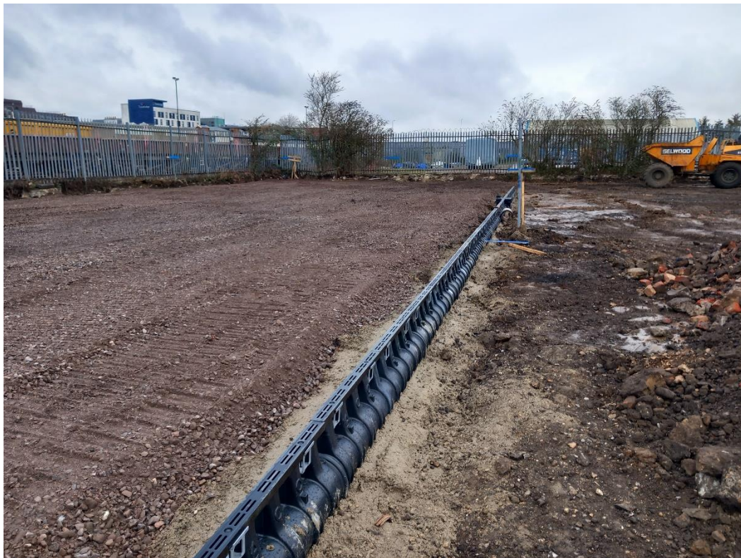
Plate 28: Site Visit 06/03/23 – Installation of surface water drainage and subbase formation levels
