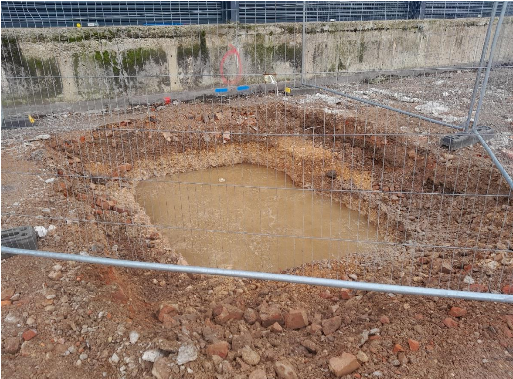
Plate 23: Site Visit 17/01/23 – Excavation for manhole chamber with rainwater and groundwater
