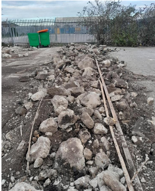
Plate 3: Site Visit 06/12/22 - breaking out of former railway track
