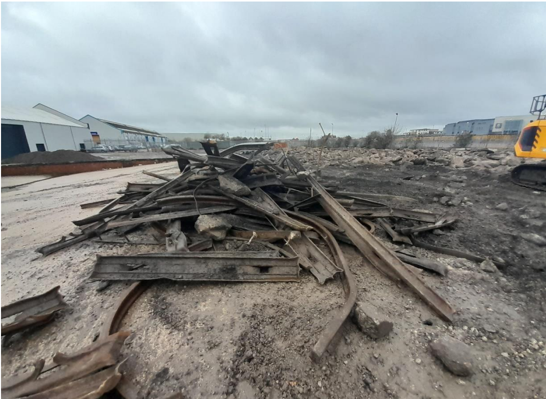
Plate 20: Site Visit 04/01/23 – Excavated railway tracks
