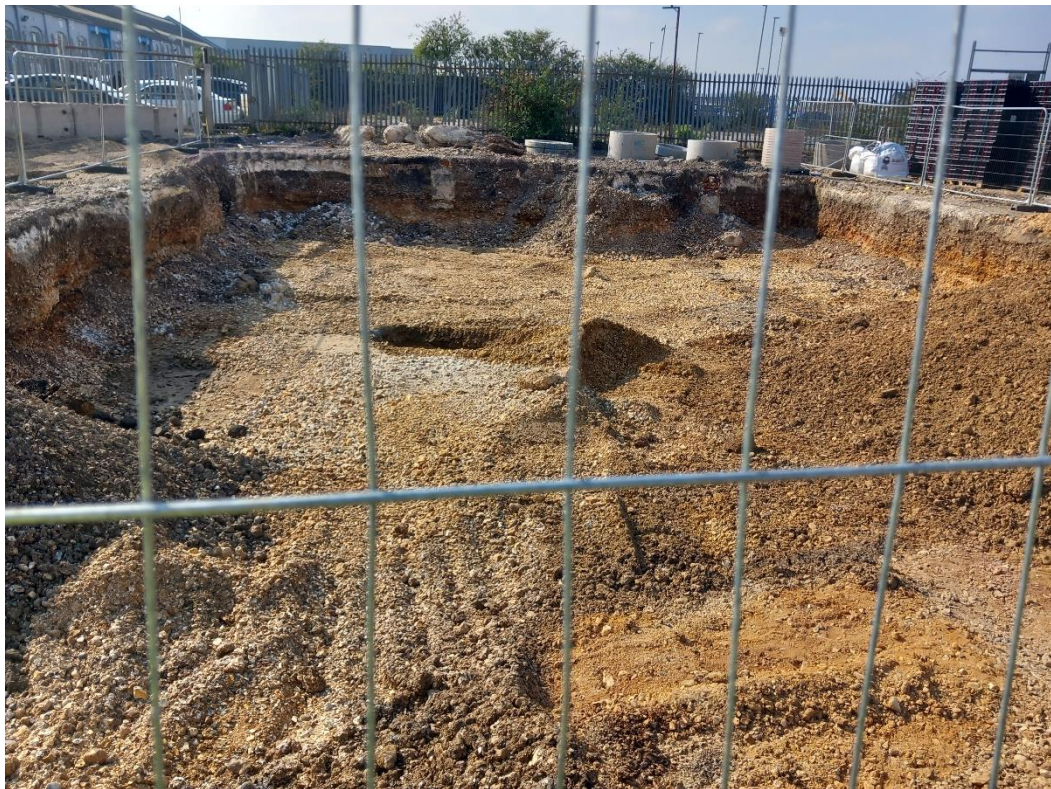
Plate 32: Site Visit 19/04/23 – Excavation for attenuation tank into natural soils
