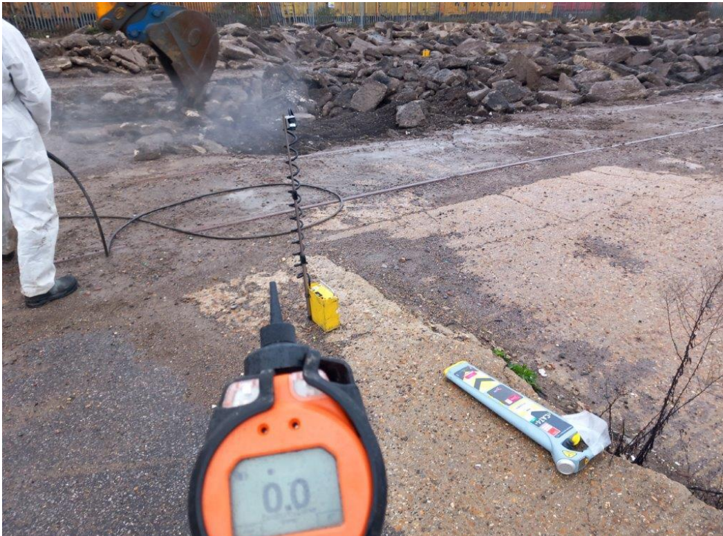
Plate 13: Site Visit 22/12/22 – VOC monitoring
