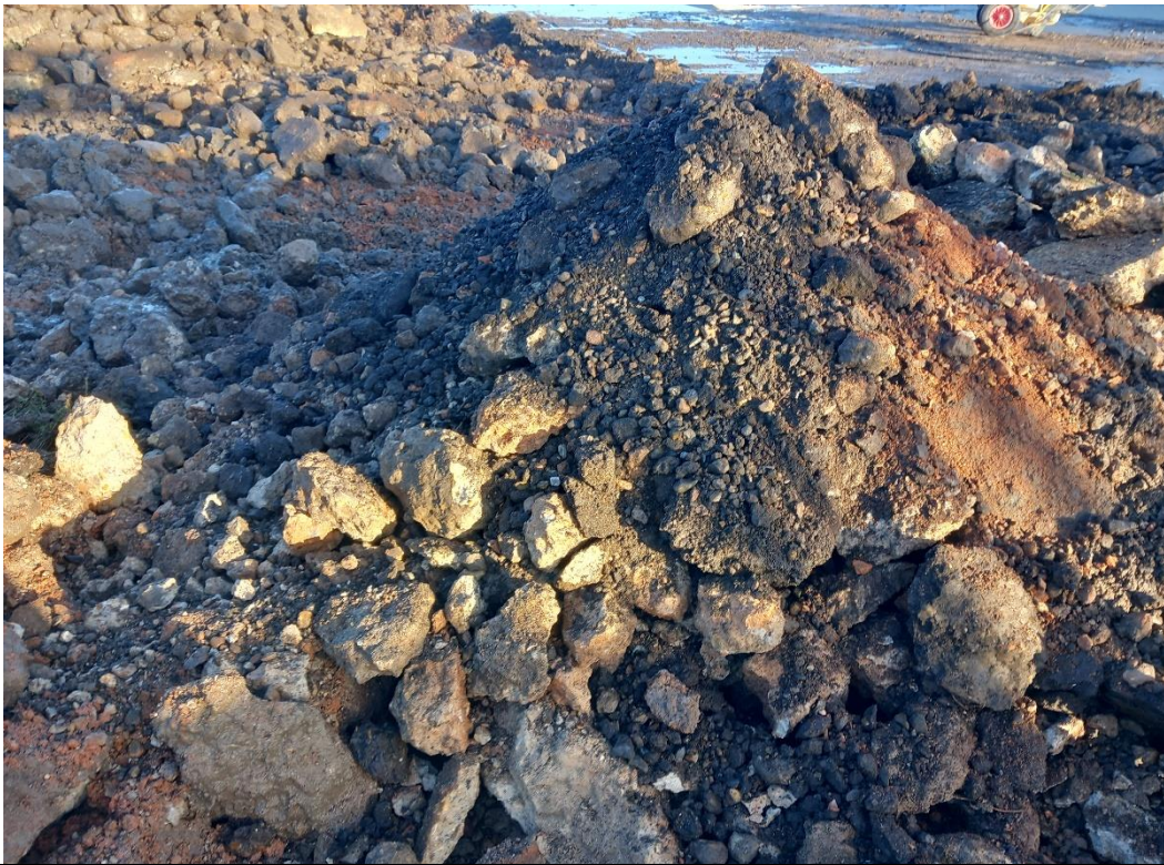
Plate 15: Site Visit 20/12/22 – General broken out material in west of the site
