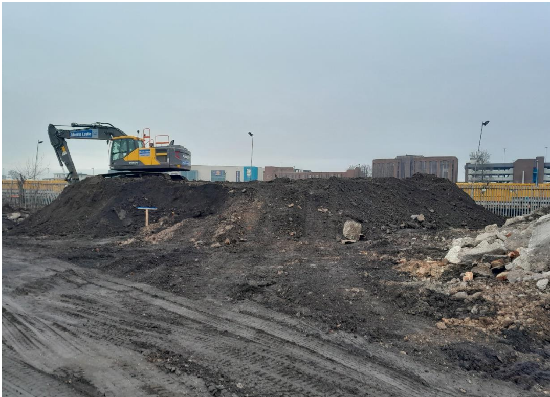
Plate 27: Site Visit 09/02/23 – Stockpile of general excavated material
