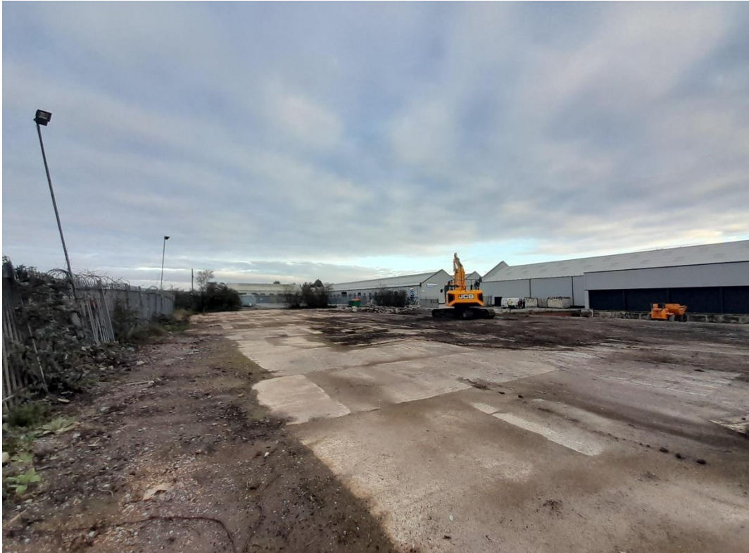
Plate 1: Site Visit 06/12/22 - Surface clearance and scraping of soft material, showing former hardstanding surfacing
