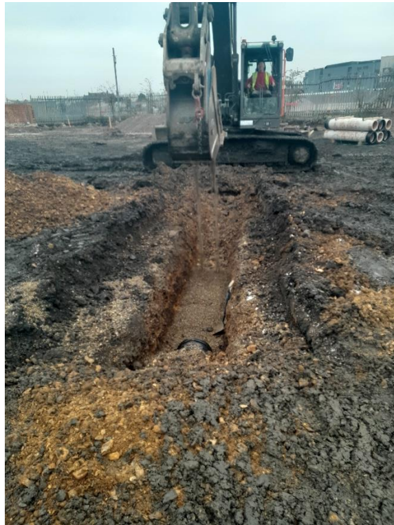
Plate 26: Site Visit 09/03/23 – Site Visit 24/01/23 – Excavation of drainage channel within natural alluvium
