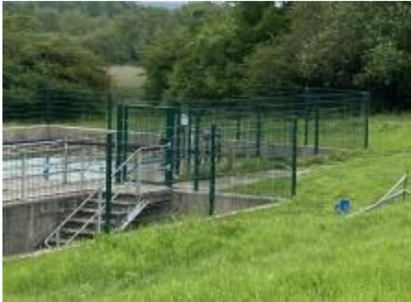
Figure 5. Treatment pool (taken May 2024)
