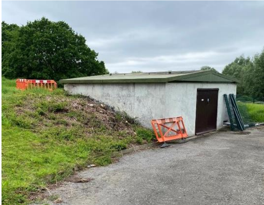
Figure 7. Single-storey building (taken May 2024).
