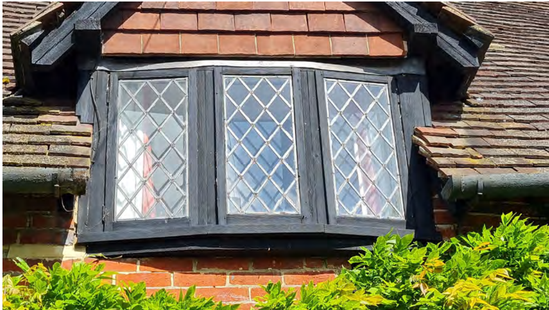
Figure 15; Close-up view of the modern bow window to the dormer. In this photo the position of the wall plate can be judged relative to the window.
