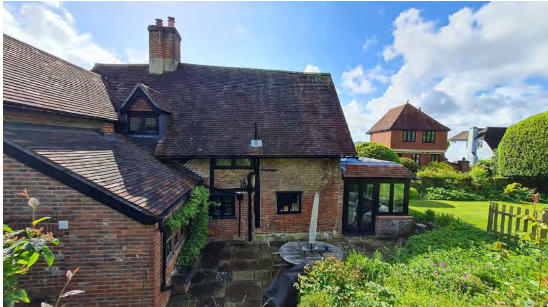
Figure 29; View of the North-West (rear) elevation of the main body of the house.
