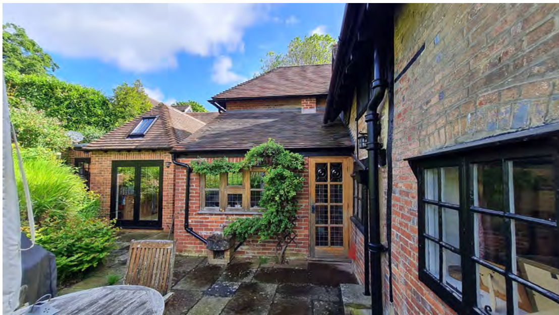
Figure 28; Closer view of the South-West elevation of the extension elements.
