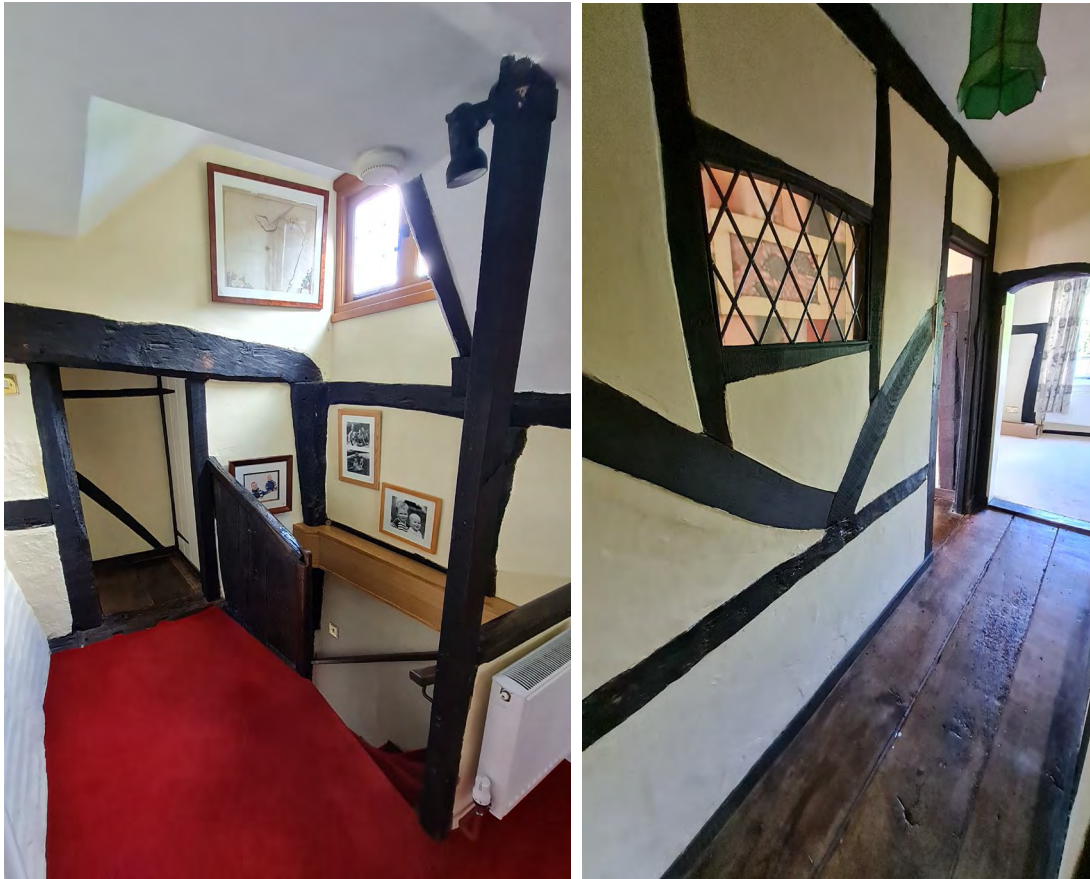
Figure 41 (left); View from the landing looking South-West, with the timber handrail and the low tie beam visible. Figure 42 (right); View along the passage formed through the central bay to the South-West of the half-bay, showing the wide floorboards and whimsical arrangement of the 'timber frame' to the later partition walls which divide the Bathroom and Bedroom. The low tie beam which has been scalloped out to improve headroom is visible at the end.
