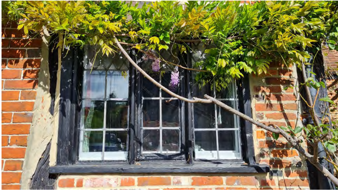
Figure 17; Close-up view of the ground floor window with the mixed lights set within steel frames to the Dining Room.
