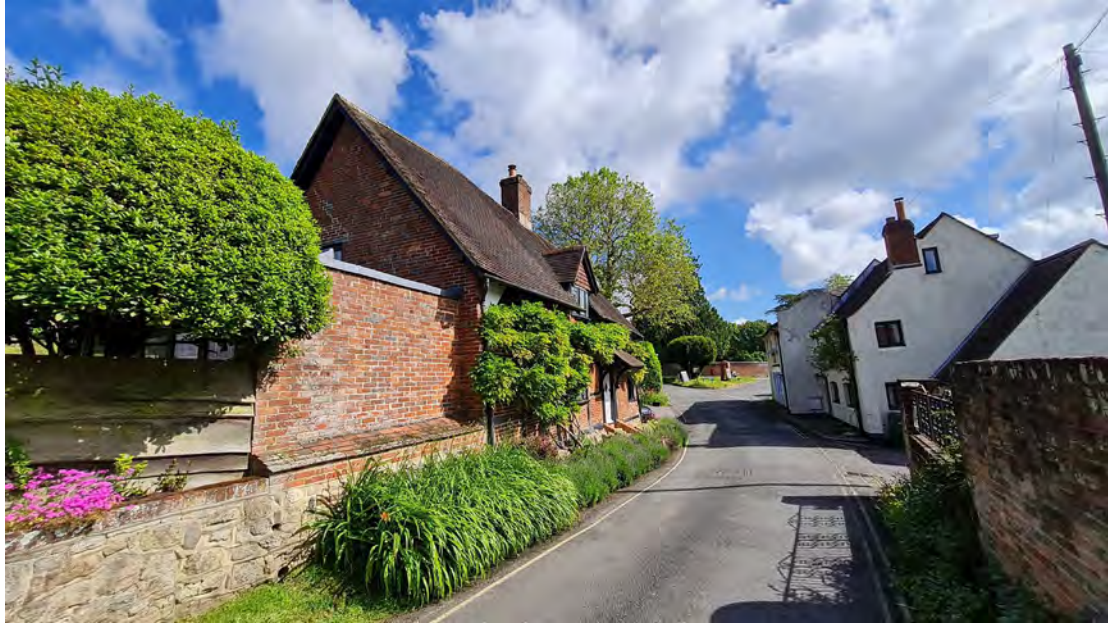
Figure 8; View looking North-East along High Street, with The Old Cottage on the left-hand side.
