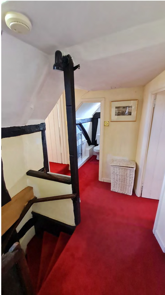
Figure 48 (left); View of the landing looking North-East. Note the lack of tie beam on the frame line (approximately to the side of the stair).
