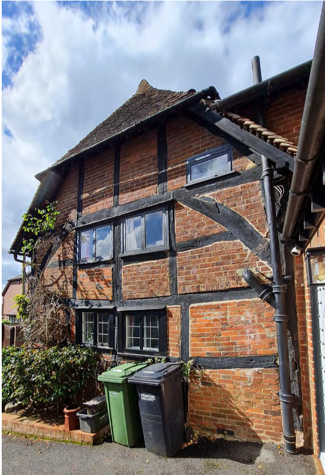
Figure 22; View of the North-East elevation from adjacent to the converted garage.
