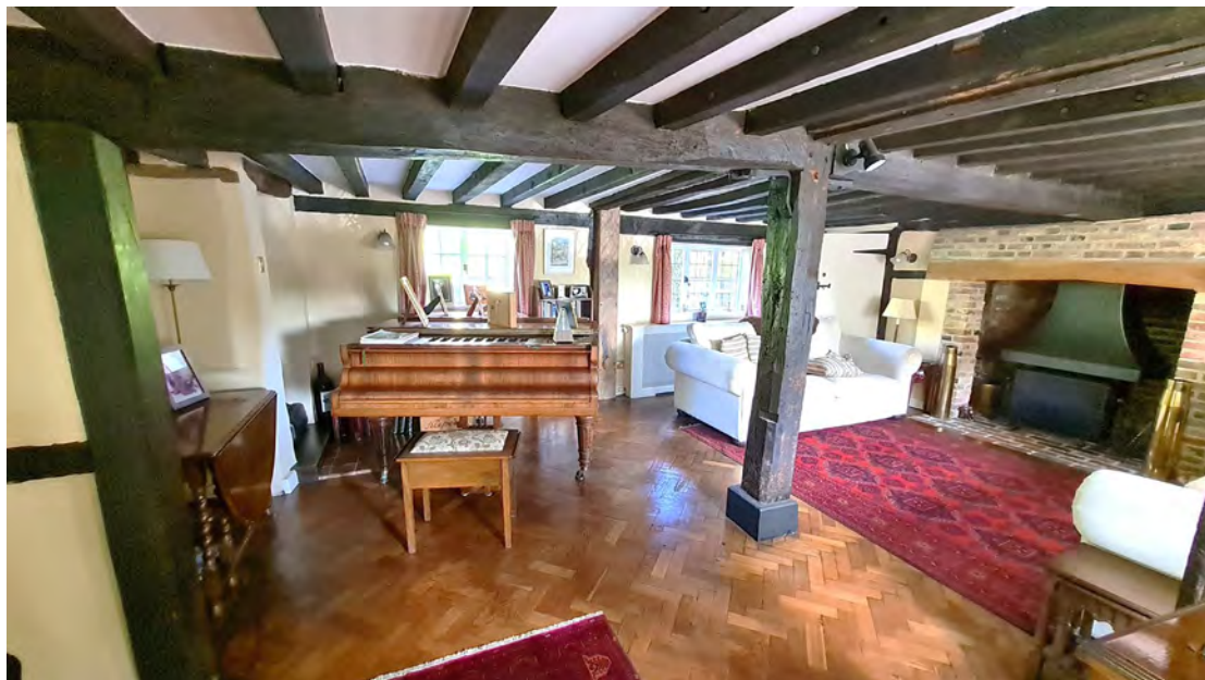
Figure 33; Image of the Living Room, showing the first-floor structure.
