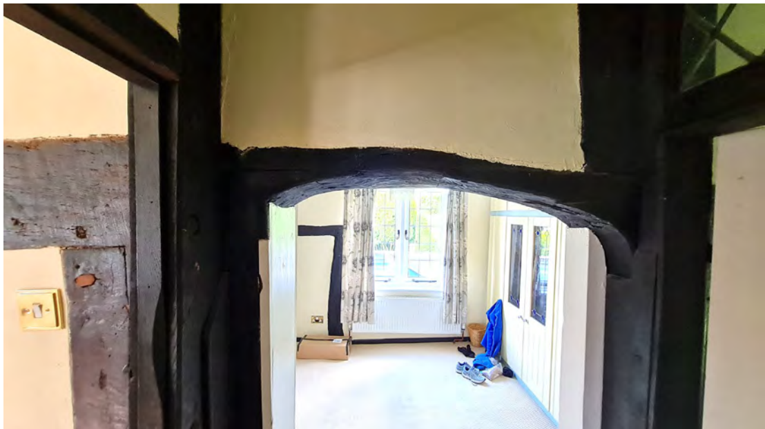
Figure 43; View of the tie beam at the doorway from the passage to the Master Bedroom. The reduction in depth to improve headroom is visible, especially when compared to the full depth visible in the adjacent Bedroom.
