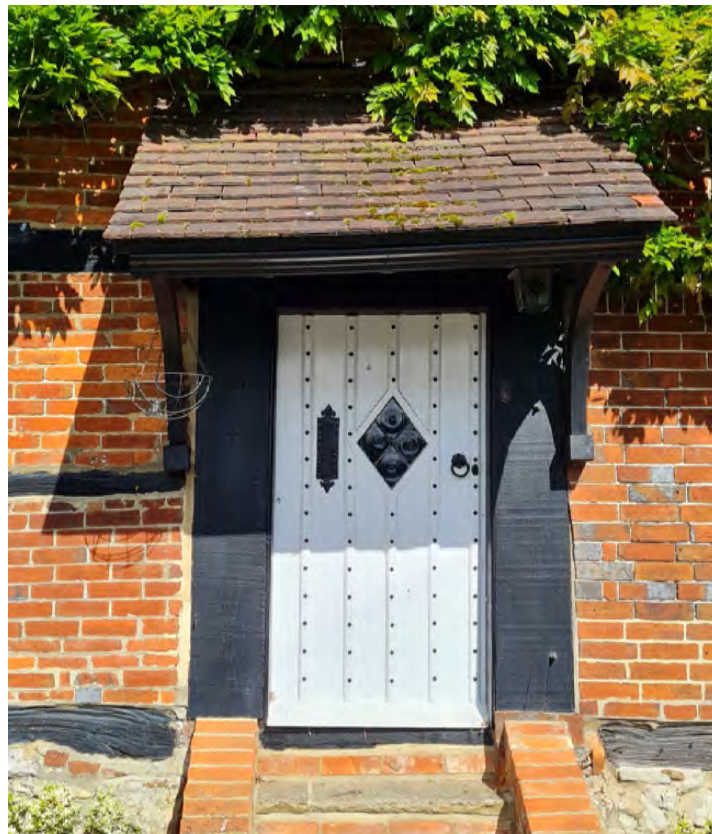
Figure 20; View of the porch. Note also the wide cover strips to each side of the door, which appear oversized.
