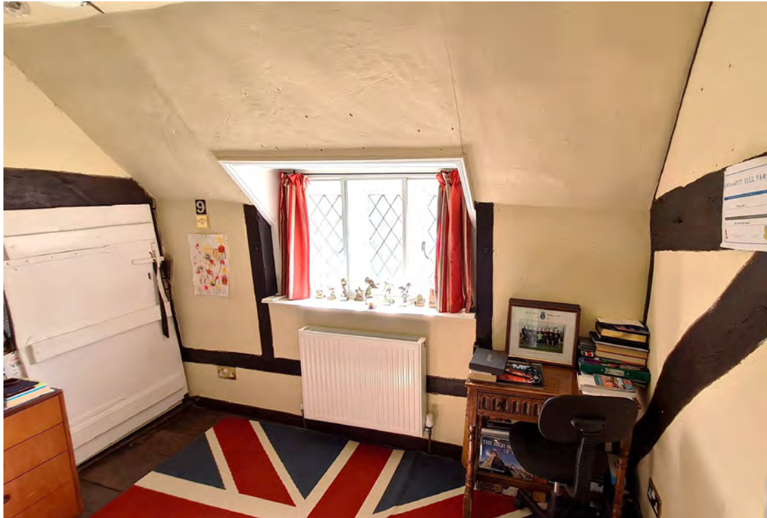
Figure 44; View of the dormer window in the Bedroom to the central bay. The line of the wall plate is apparent from the position of the skilling and the intersection of the tie beams to the frames as they intersect the external walls. The door to the half bay 'lobby' space on the first floor is visible to the left.
