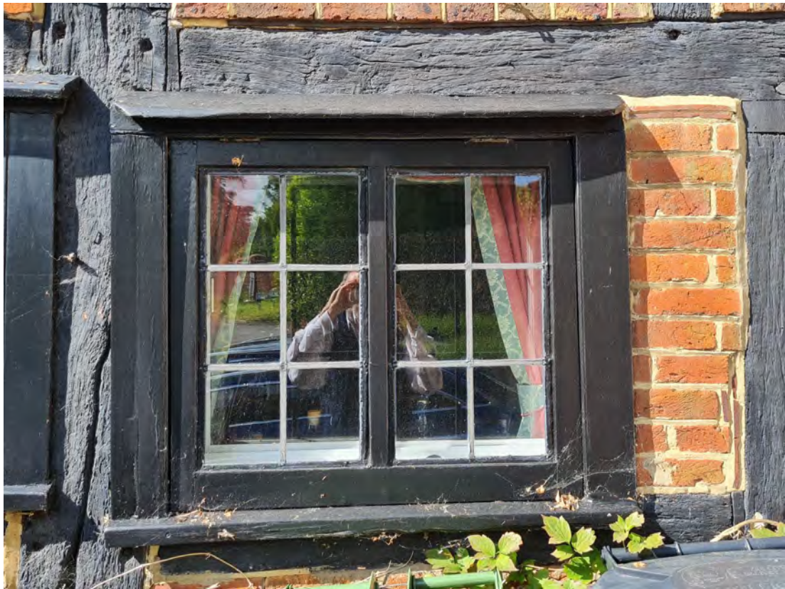
Figure 24; The right-hand of the ground floor windows to the North-East elevation, showing the modern top-hung casement.
