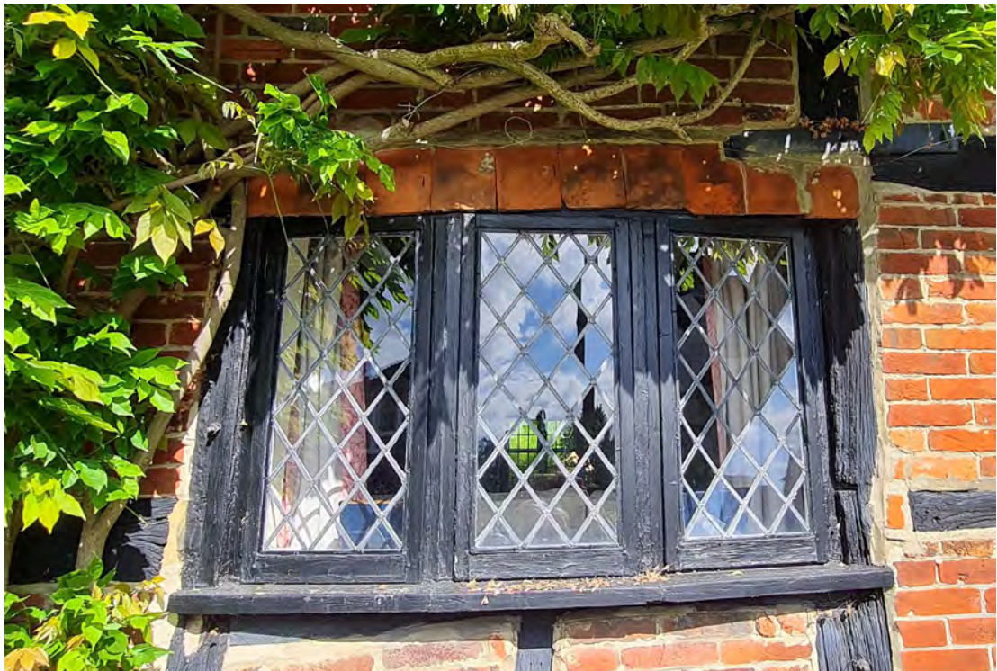
Figure 16; Close-up view of the modern bow window to the Living Room.
