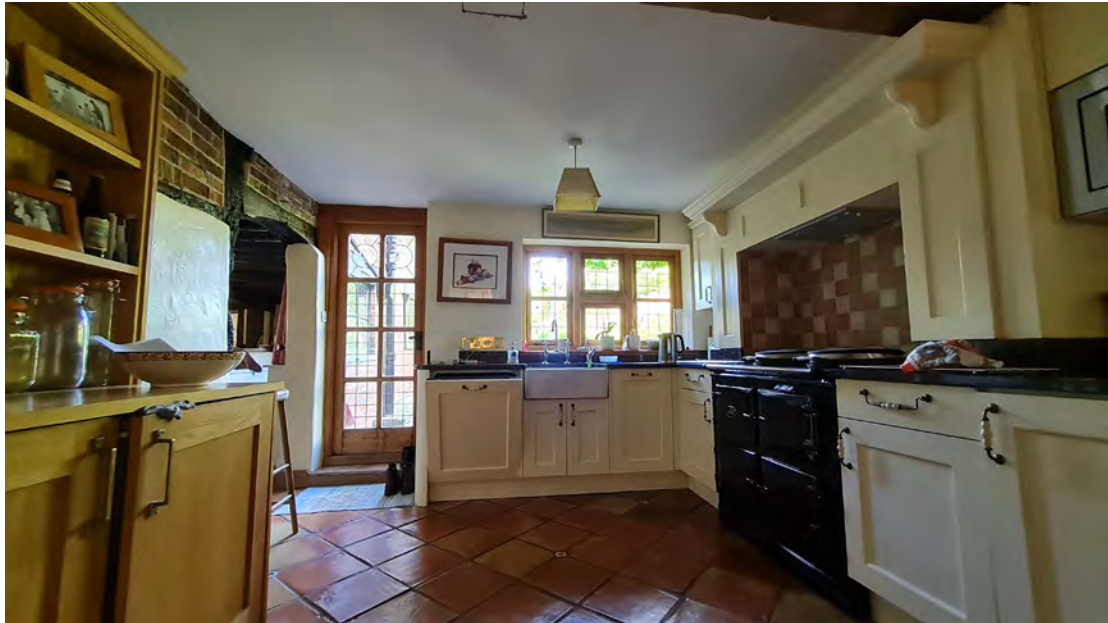
Figure 38; View of the Kitchen looking South-West, toward the external door leading to the terrace. The apparent fireplace containing the range cooker is in fact modern false-work.
