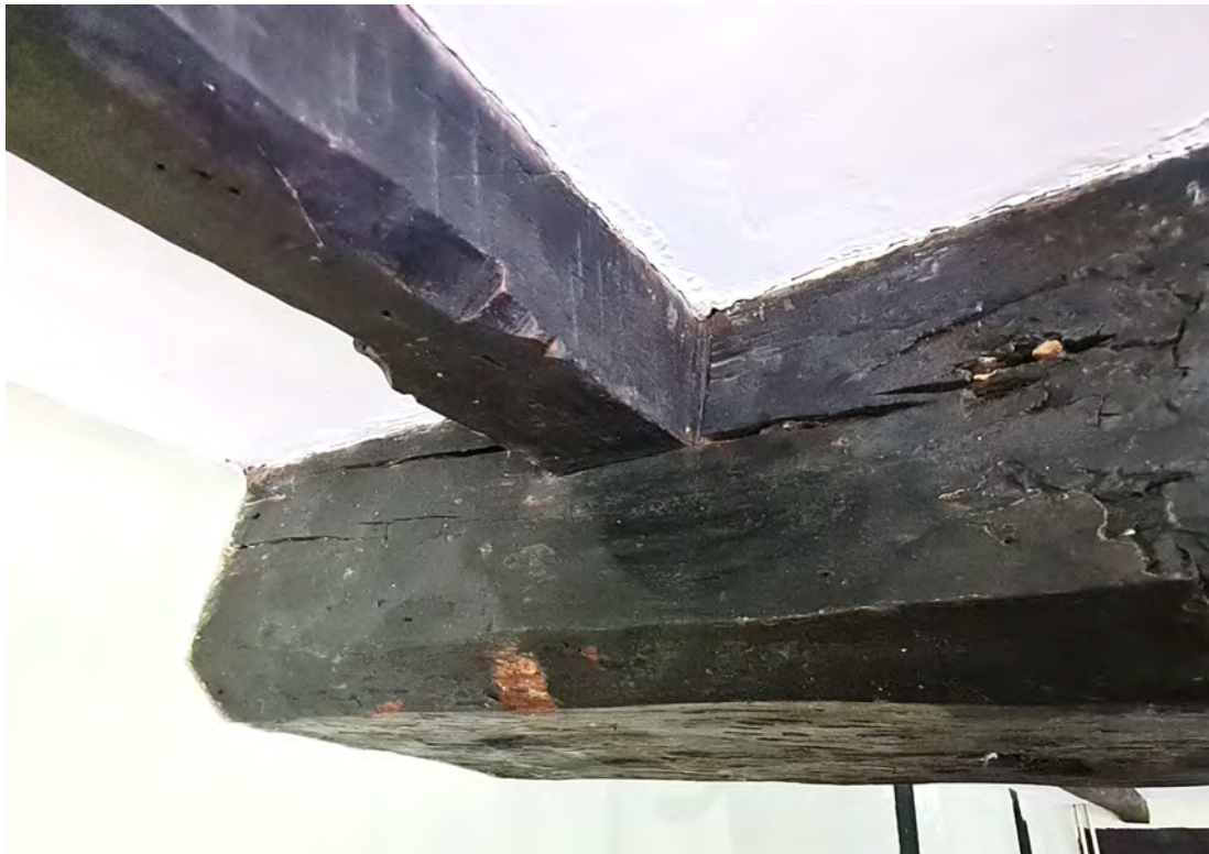
Figure 37; View of the axial beam, unstopped, and a floor joist, stopped with a curved step-stop and nick, to the Dining Room.
