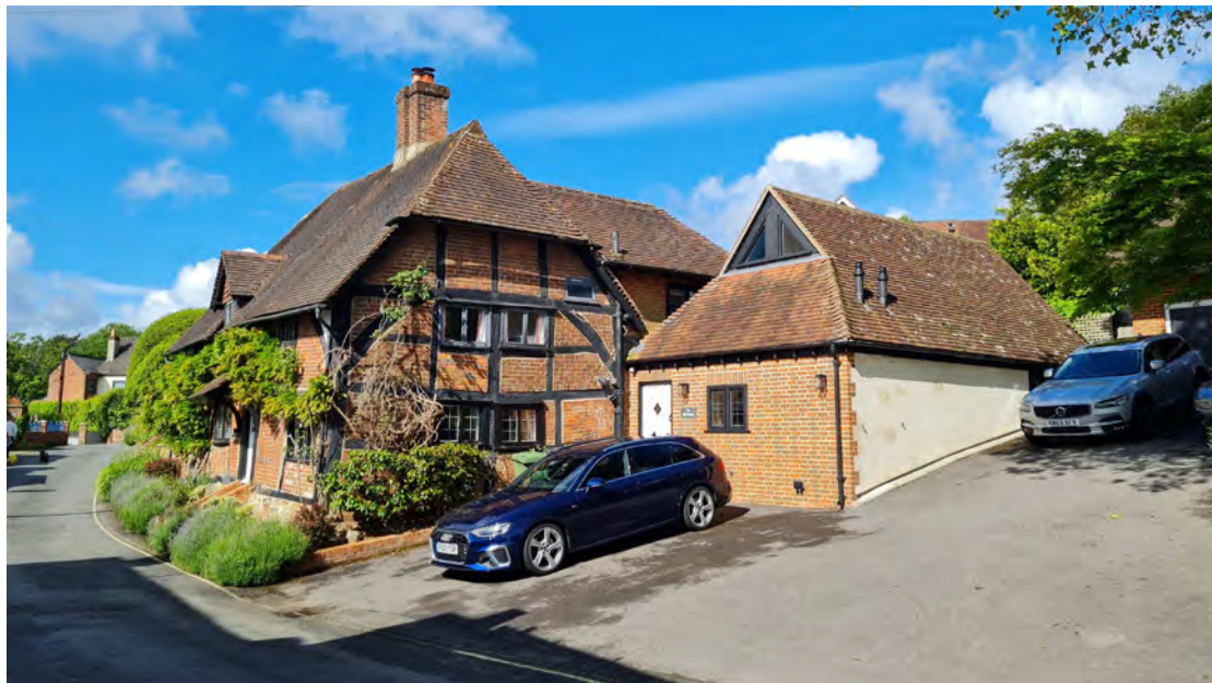
Figure 21; View of the North-East elevation as seen when coming along High Street. The set-back of the converted garage allows the observer to appreciate the age and character of the building.
