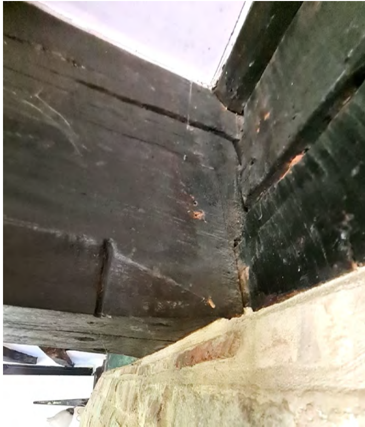
Figure 34; Image of the step stop to the end of the primary floor beam in the Living Room where it meets the masonry of the chimney above the fireplace.
