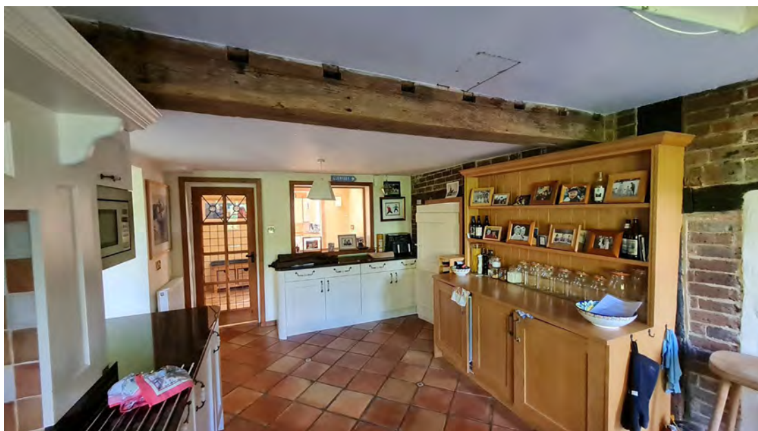
Figure 40; View Kitchen looking North-East toward the current entrance hall. Note the reclaimed beam in the ceiling. The door back through to the Dining Room is in the background, on the right, also passing under the floor girt, which continues again to the bay passed the stair.
