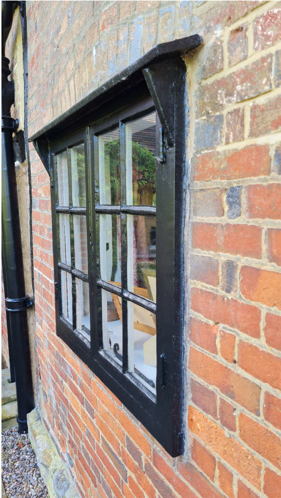
Figure 31; Image to show a close-up view of the frame sitting outside the face of the wall.
