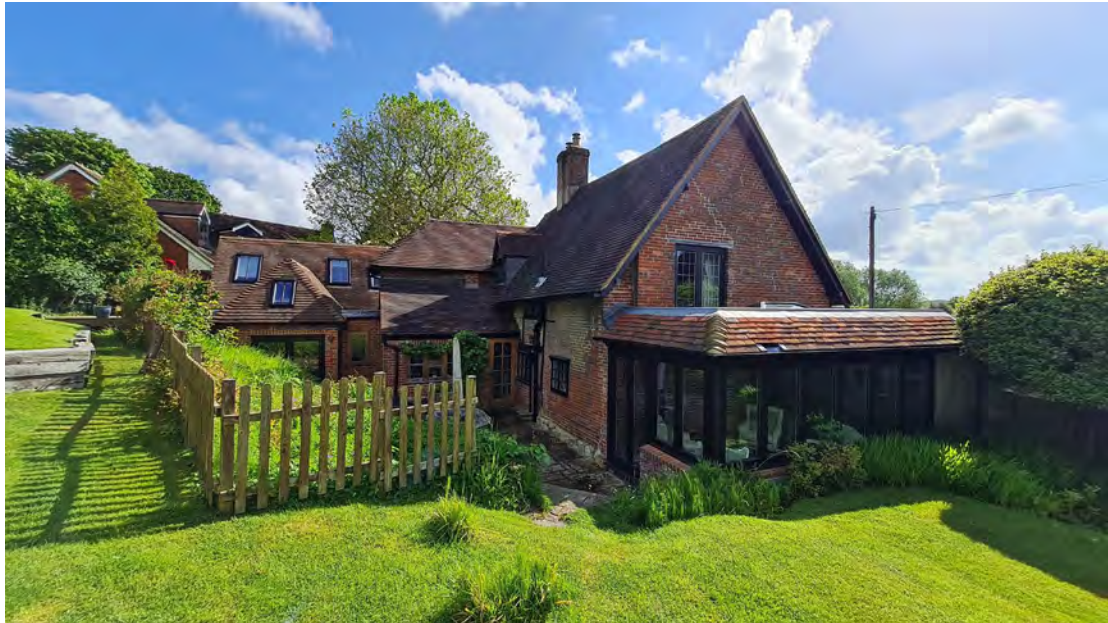
Figure 27; The South-West elevation, with the two-storey element of the original cottage and modern conservatory in the foreground, and the mixture of extensions to the original house set back behind.
