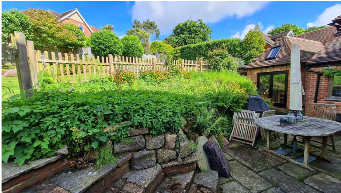
Figure 32; Image to show the current retaining structure and bank.
