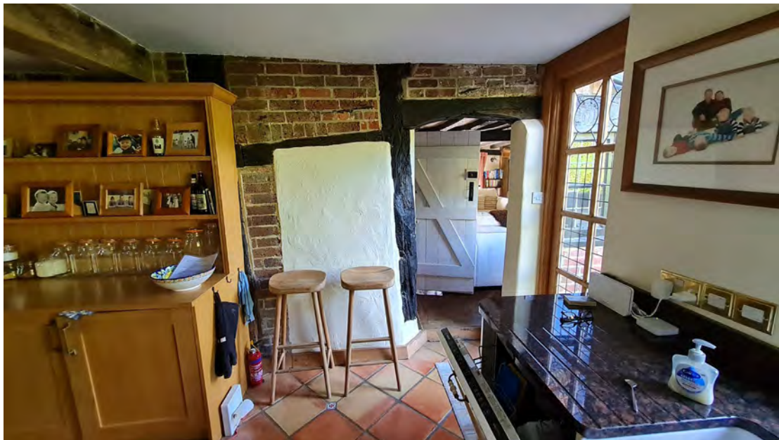
Figure 39; View Kitchen looking South-East toward the dividing wall which was once the rear external wall of the cottage.
