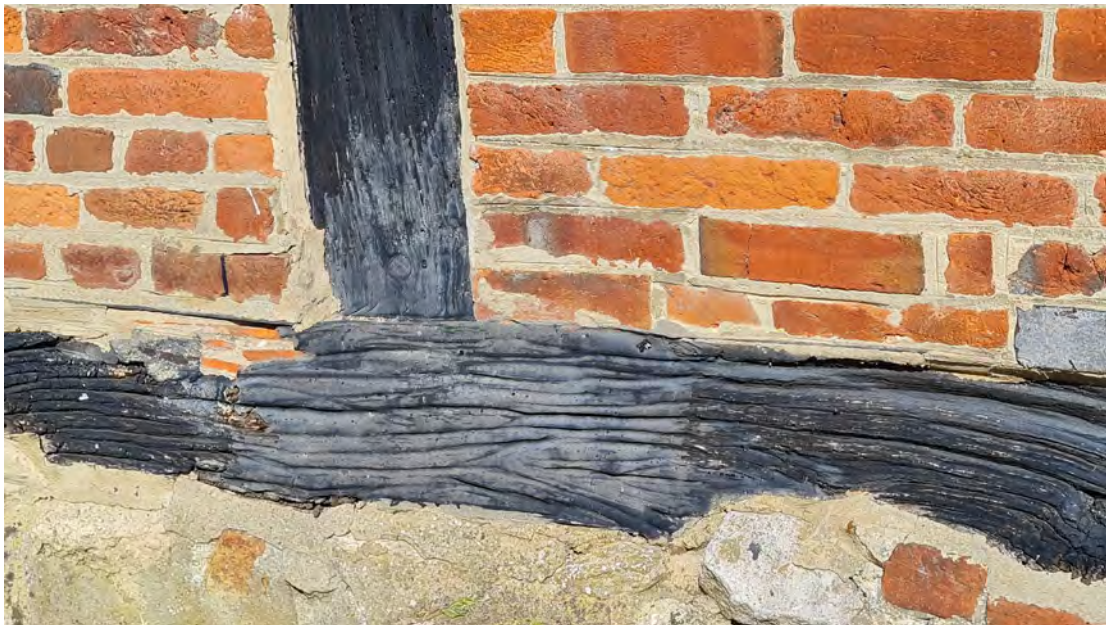
Figure 13; Close-up view of a section of cill beam, with the resin repair to the cill and lower section of the post clearly visible, despite the attempt to disguise this with fake 'grain'.
