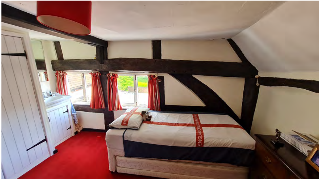
Figure 51; View of the North-Eastern end wall in the Bedroom, with the timber frame and curved brace visible, together with the unattractive late twentieth century windows.
