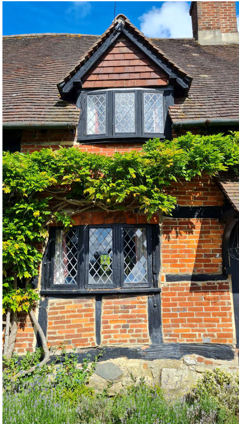
Figure 11; View of the bay of the South-East elevation which contains the dormer. Note also the tiles covering the floor girt above the ground floor bow window.
