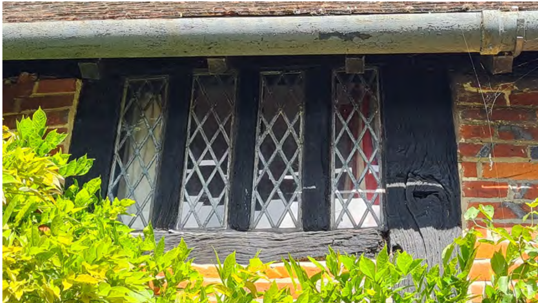
Figure 18; Close-up view of the interesting, mullioned window to the first floor, which serves the North-Eastern bedroom. This retains something of a late medieval or early modern window, and is significantly more pleasing to the eye than the others to this elevation.
