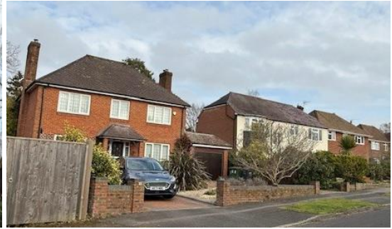
Image 3: Two storey houses to the rear at 20/22 Grosvenor Road
