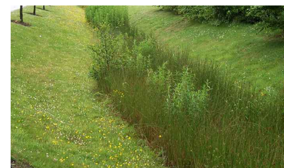
Newly formed swale
