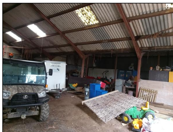
Photo 4 Interior showing polycarbonate sections to roof
