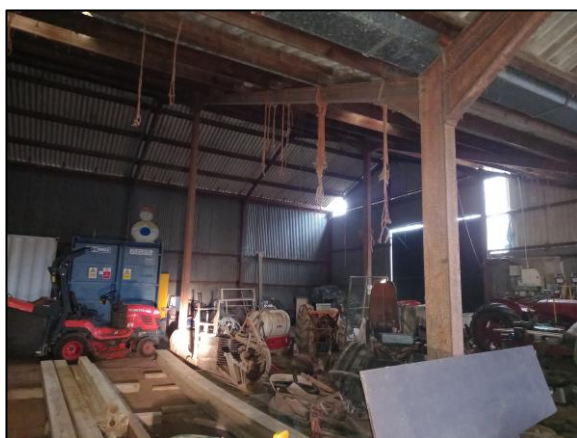
Photo 3 Interior showing steel frame and stored materials
