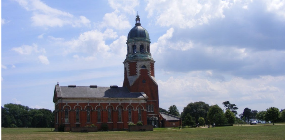
Figure 4 - The North West Elevation of the Chapel showing the former toilet block.
