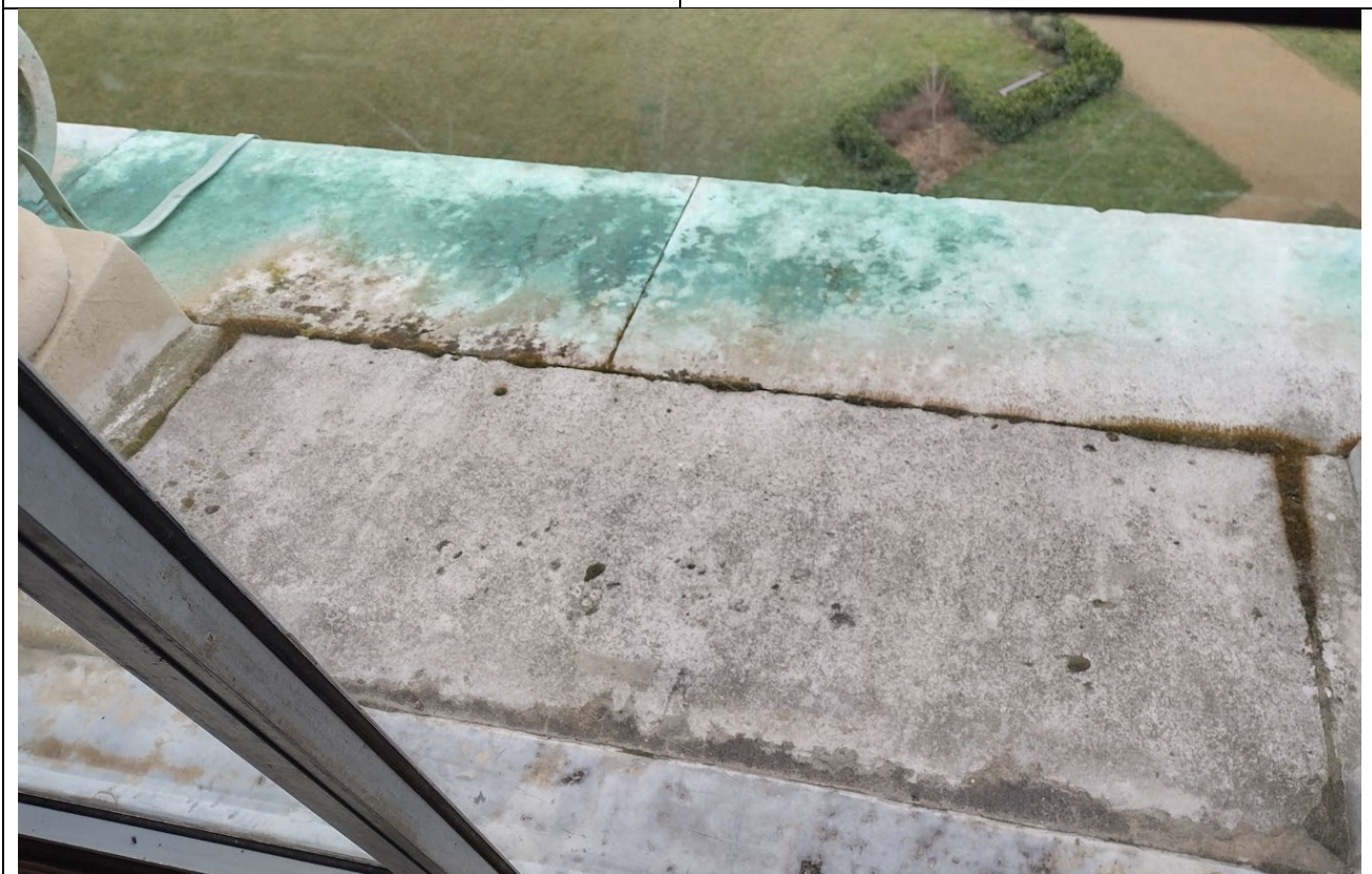
Fig 22 Upper stonework pointing, and leadwork
