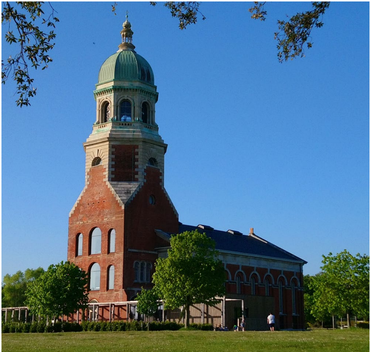
Figure 2 - The Chapel tower and the recently added café and pergola.
