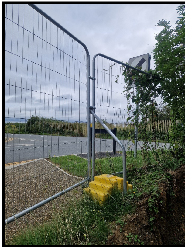
Plate 3: Low-level tree protection barriers.
