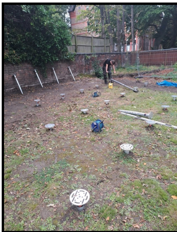
Plate 1: Hand-driven piles to support a ring beam.
