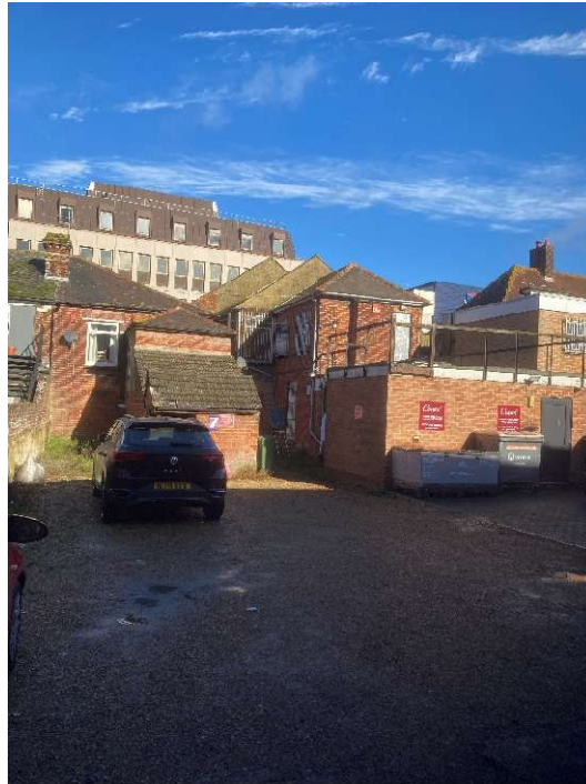
Fig. 3 – Photograph showing the rear (south) elevation of 5 Leigh Road with the existing balustrade shown around the balcony area at first floor level and the bin storage at ground floor level.
