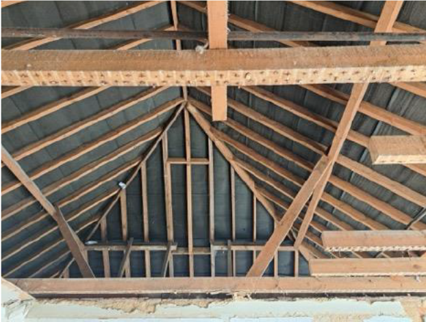
Photograph 1. Internal roof space at 2 Western Road.
