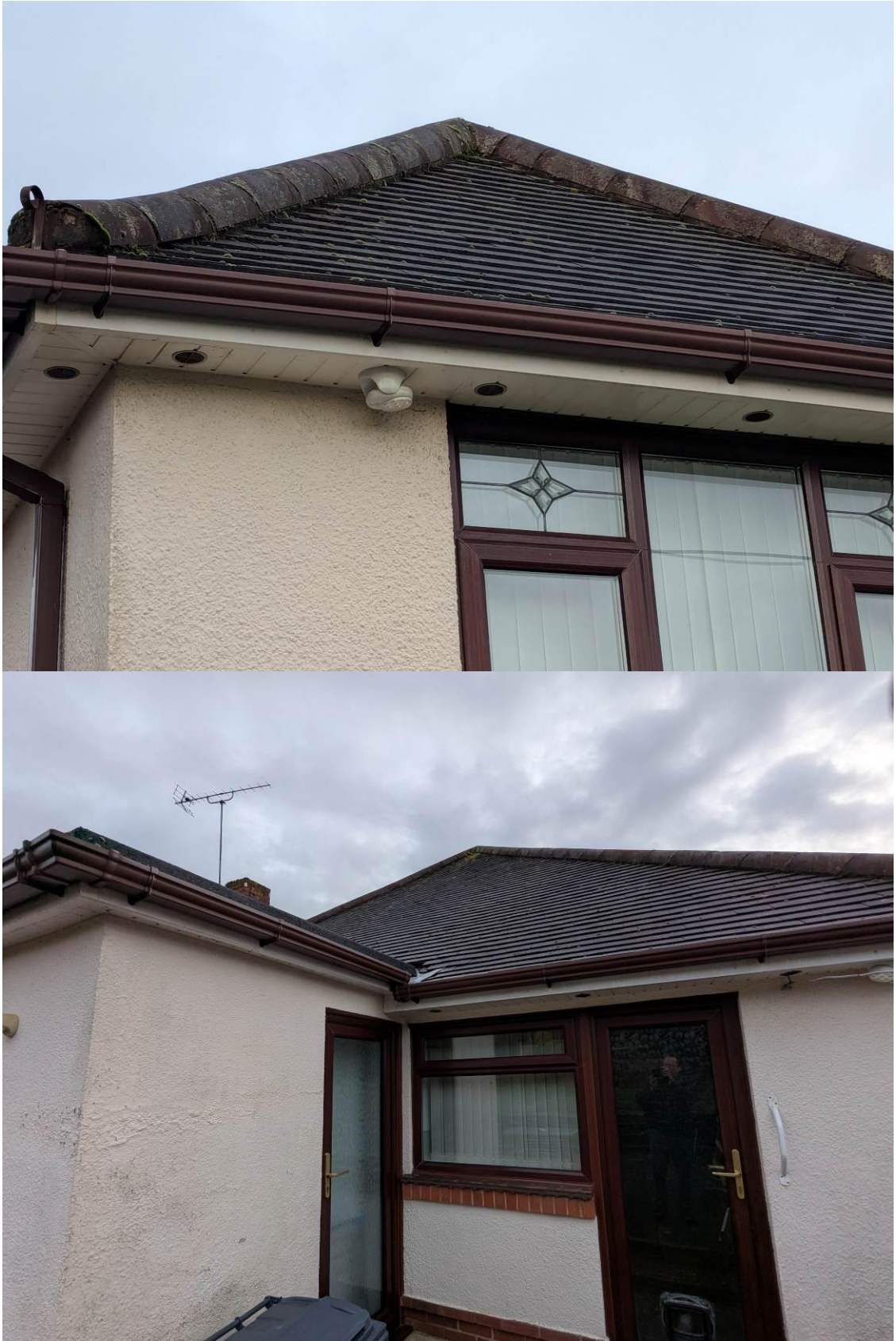
Photo 3/4 22 Trevoise Crescent, (east and west aspect)roof detail
