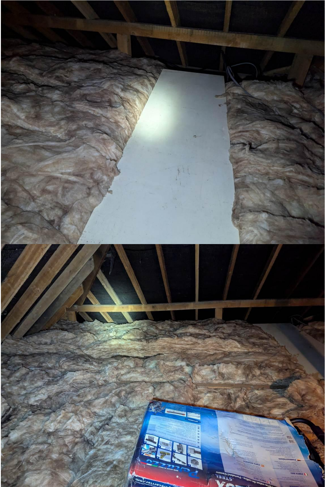
Photo 11/12 Internal area roof areas fully inspected. No Dropping or other evidence of bat use recorded.
