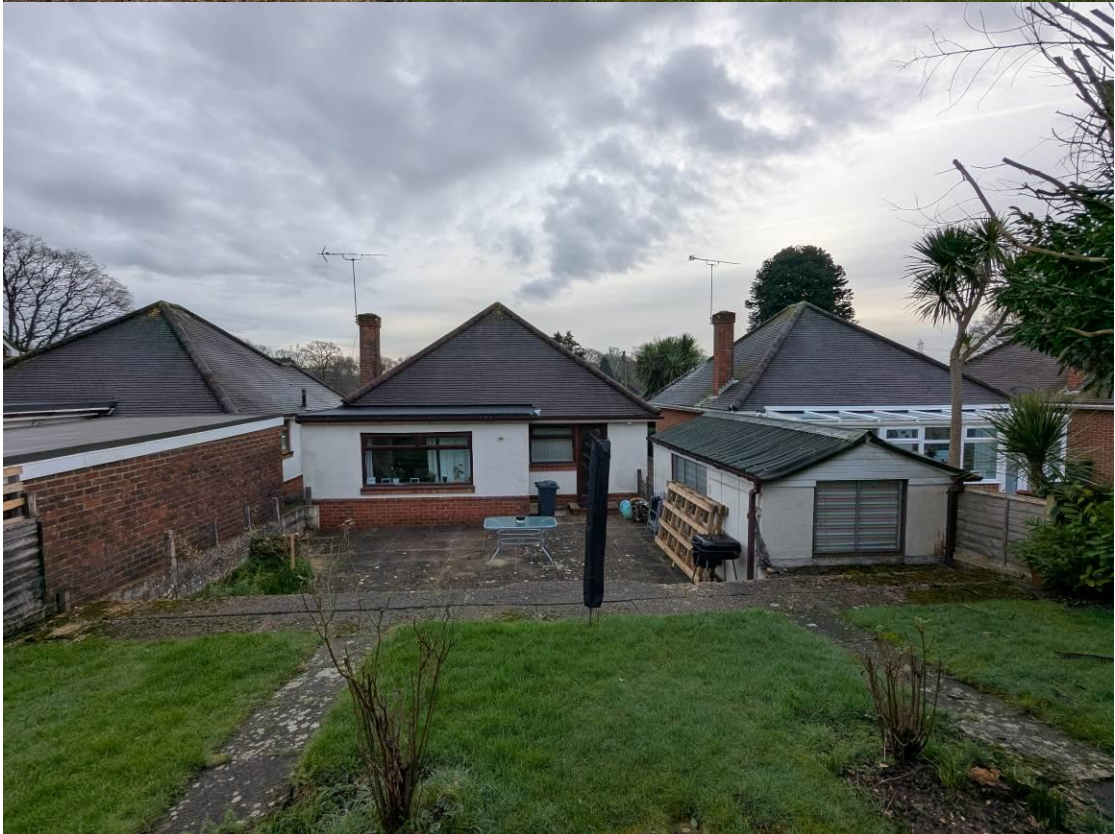
Photo 1/2 22 Trevoze Crescent (east and west aspect)
