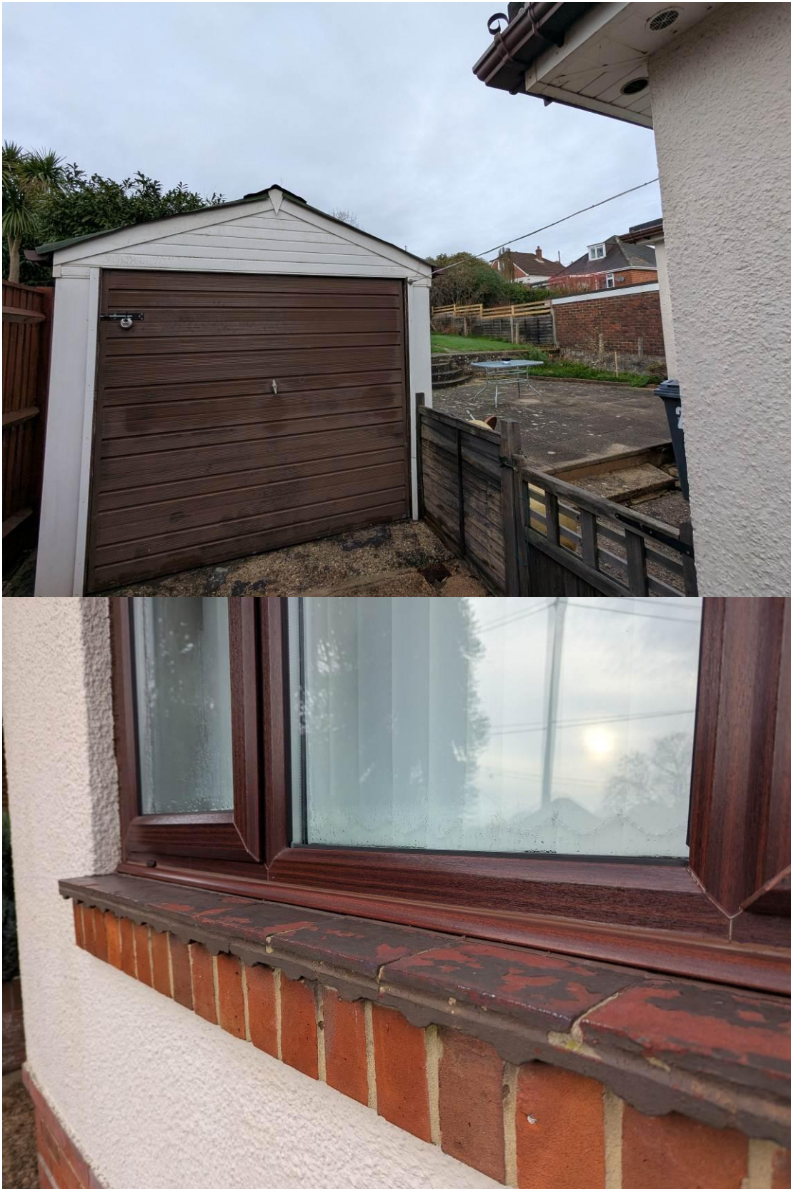
Photo 7/8 22 Trevoise Crescent– east aspect -.. No droppings or evidence of use internally or externally.
