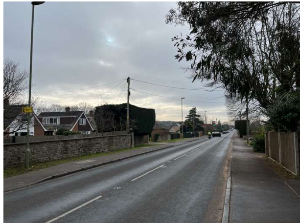
The approach to the site from the north, on Botley Road.
