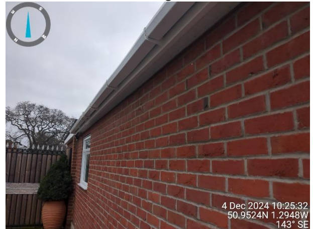
Photograph 4: View of the bungalow soffits which are in good condition and flush with the wall.
