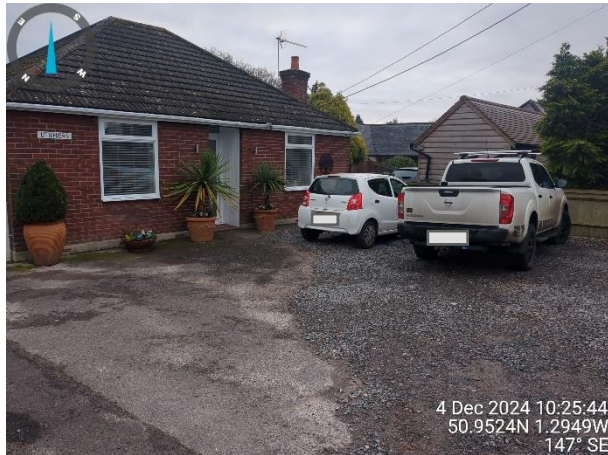
Photograph 1: View of the front of Littledean bungalow.
