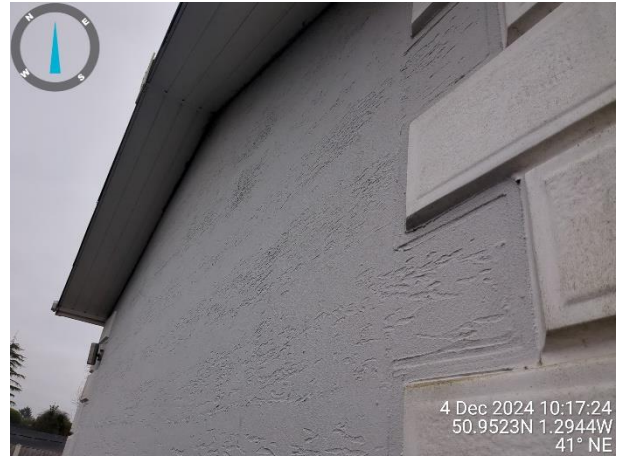
Photograph 14: View of mobile home gable, which is absent of gaps, due to nature of its design.
