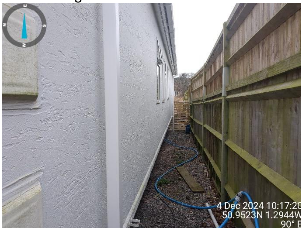
Photograph 15: View of the rear of the mobile home with hardstanding only present.
