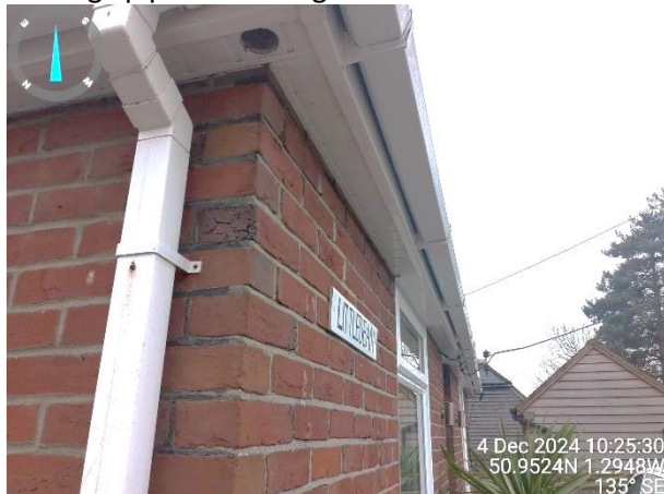
Photograph 5: View of the soffits at the front of the bungalow in good condition and flush with the wall. Circular hole is a vent.
