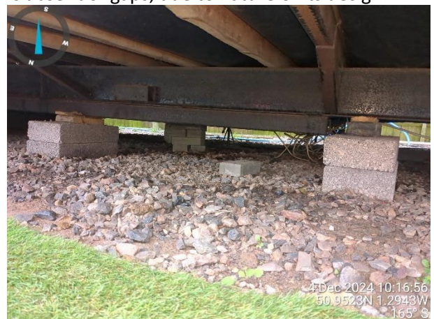
Photograph 16: View of underneath of mobile homes, with no evidence of utilisation by small mammals.
