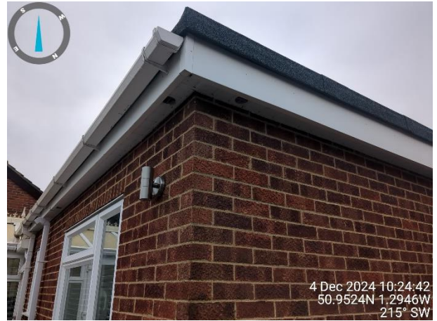
Photograph 8: View of the flat roof extension with soffits in very good condition and flush with the wall and vents present in the corner.
