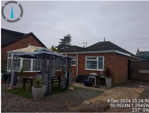
Photograph 7: View of bungalow rear with roof in very good condition and surrounded by hardstanding.
