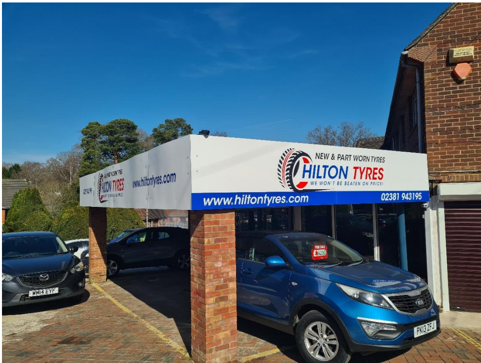
Side Elevation: Signage (as installed)
