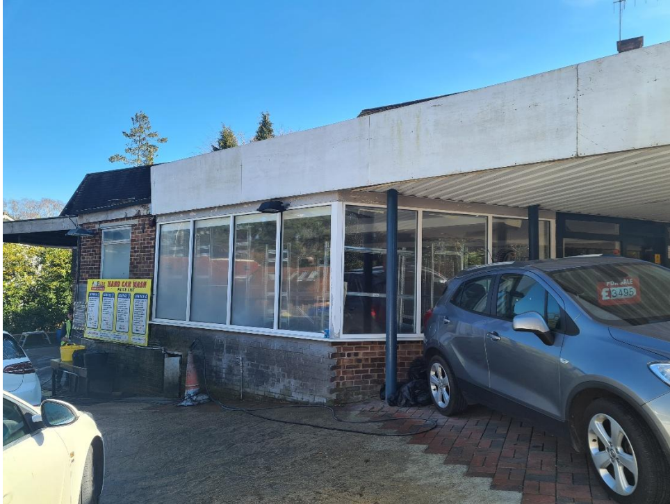
Side Elevation: No signage installed
