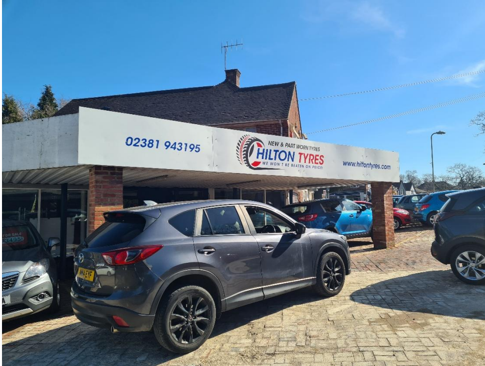
Front Elevation: Signage (as installed)
