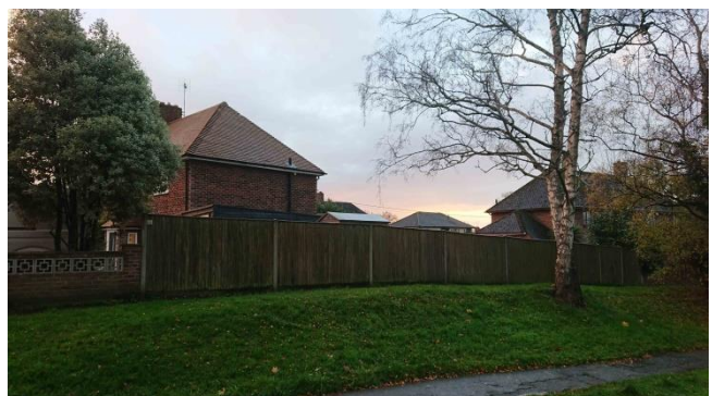
View of the side (North) elevation from Mortimers Lane (B3037) looking South West.
