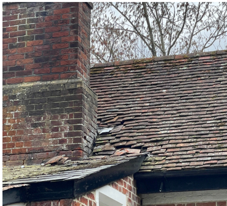
Image 5 - Key Repairs - Window 8, Slipped Roof Tiles, Internal Damp
