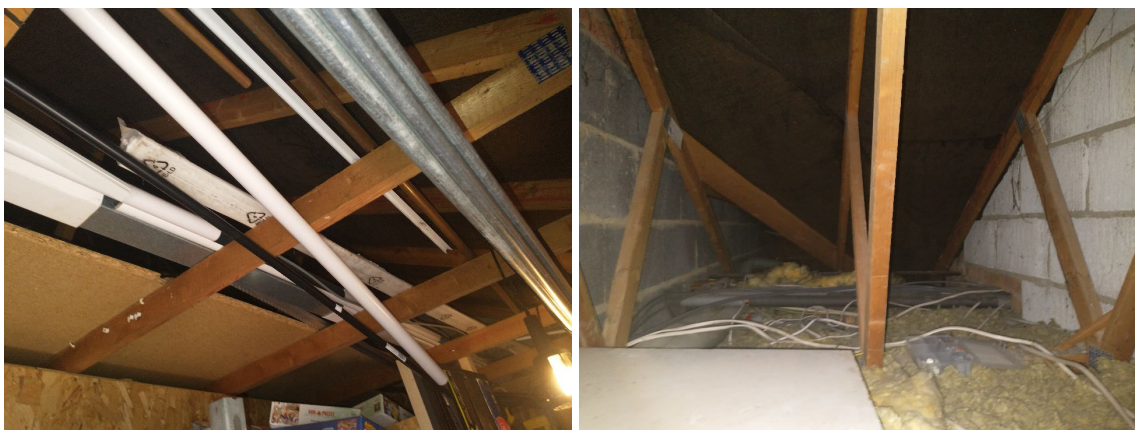
Figures 3 and 4: Open section of void over garage and smaller roof void, respectively.
