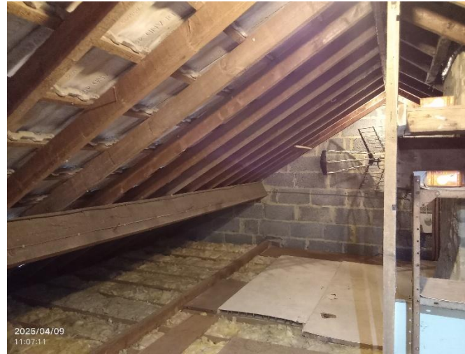
Photo 5: Internal loft void of house.
