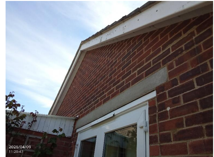
Photo 3: Rear gable end.
