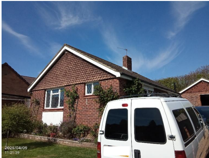
Photo 1: Front and side elevations of the building.
