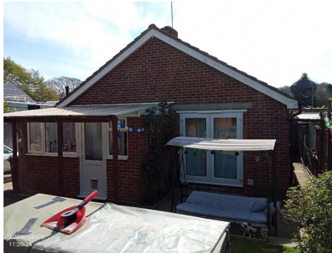
Photo 2: Rear elevation of the building.
