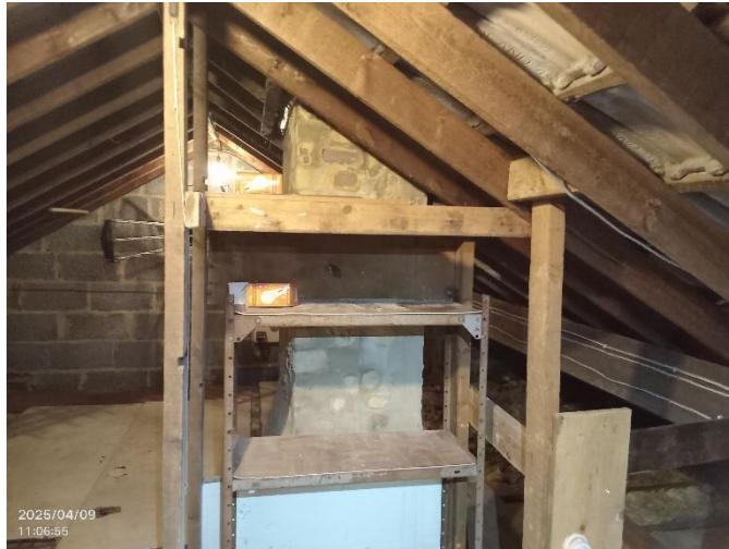
Photo 7: Internal loft void of house.
