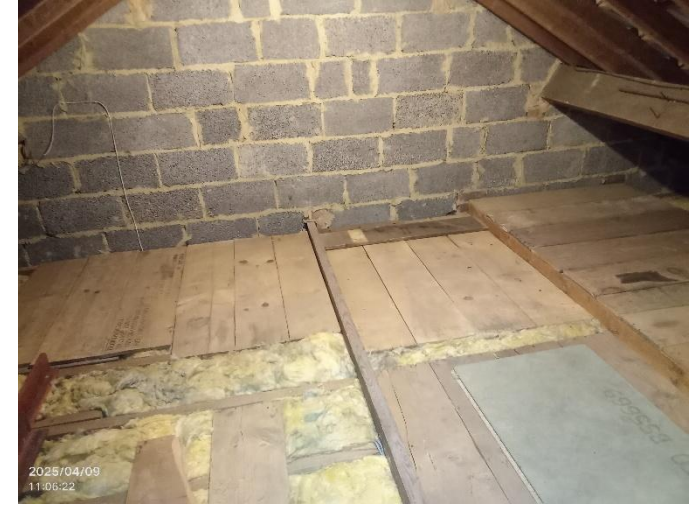
Photo 6: Internal loft void of house.
