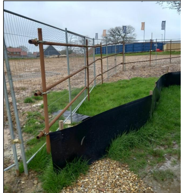
Photo 10 Site compound and reptile fencing
