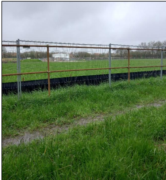
Photo 9 Reptile fencing around site
