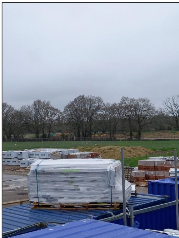
Photo 1 General view of site and compound (April 2023)
