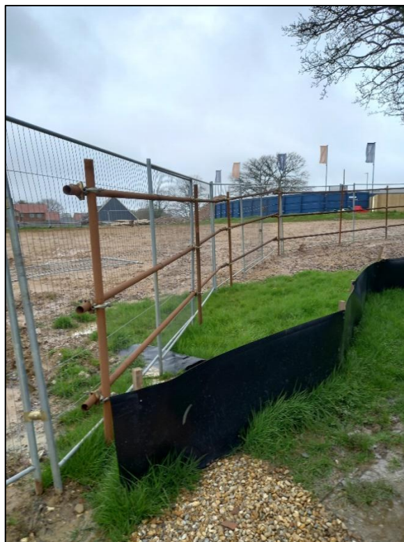
Photo 10 Site compound and reptile fencing
