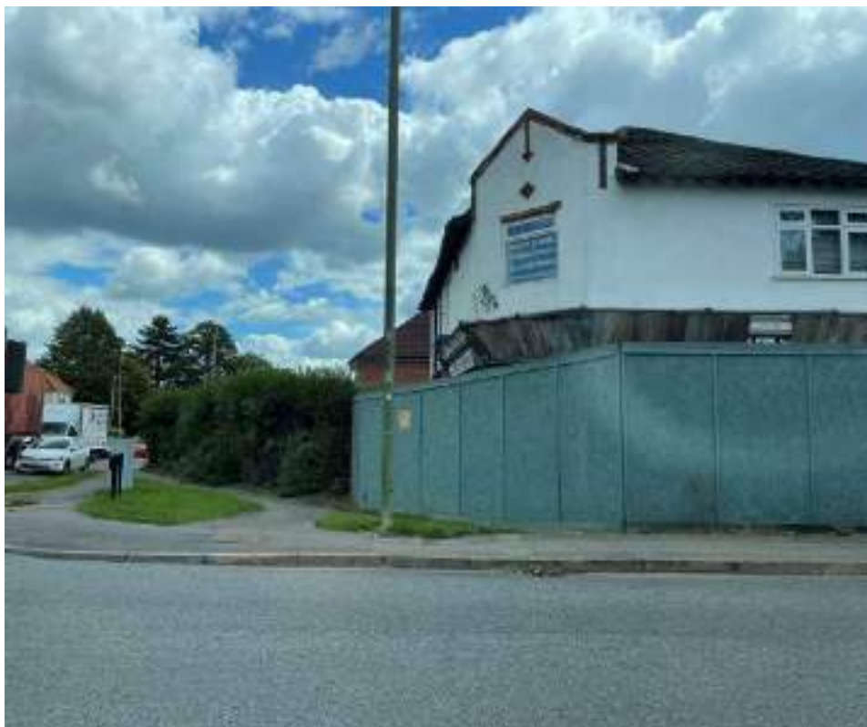
Facing east from Bournemouth Road towards the frontage of the disused commercial premises.
