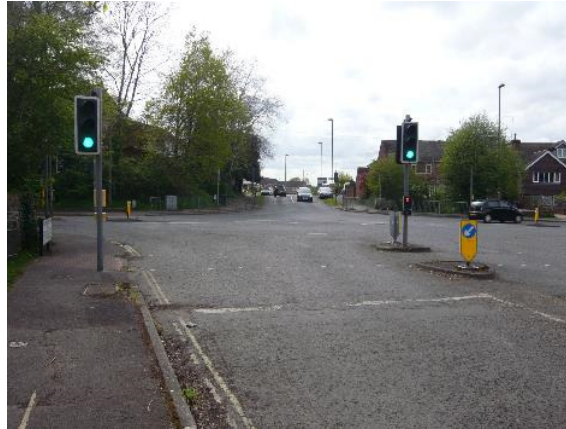
View of existing Stubbington Way approach and use of refuge for signalling equipment.
