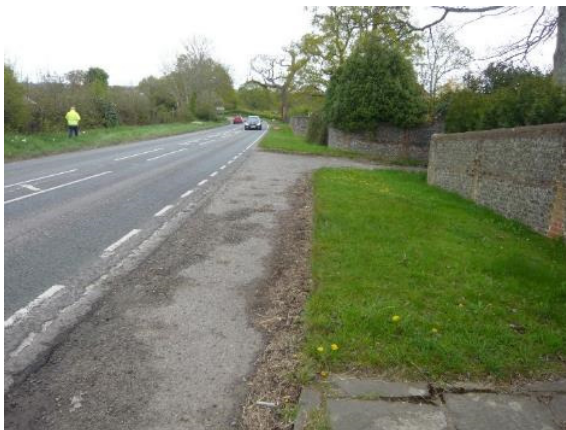
Photo G: View looking east across existing access (proposed footway link to be provided to the right of the short merge taper.)
