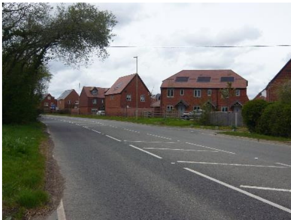
Photo A: View looking west towards existing access to Little Dower House.
