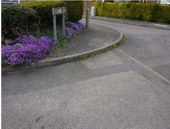
Photo C: View towards pedestrian access to existing footway on Noyce Drive.
