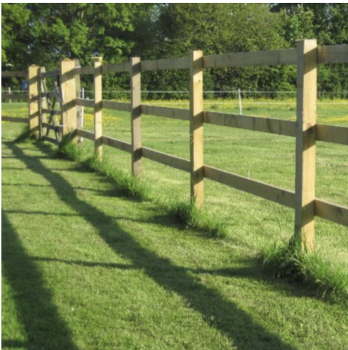
Example of Post and Rail Fence
