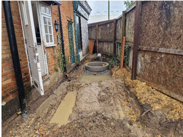
Print 6 View of drainage being constructed
