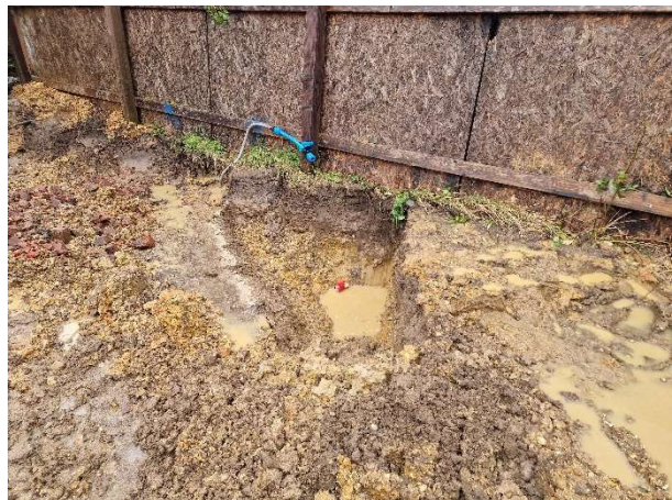
Print 4 View of an excavation
