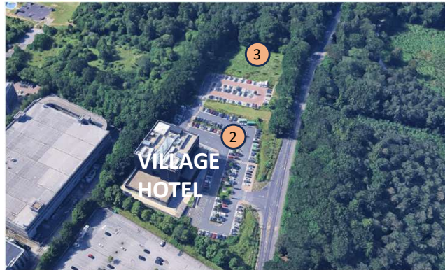
AERIAL VIEW OF HOTEL AND CAR PARK WITH PROPOSED COURTS AREA BEYOND
