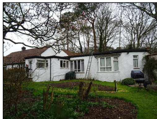
Figure 4 – flat roof extension extending from the northern end of the house
