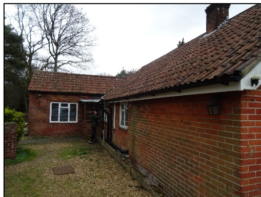
Figure 1 – south western corner of the house with the pitched extension extending from the northern elevation of the main section of house
