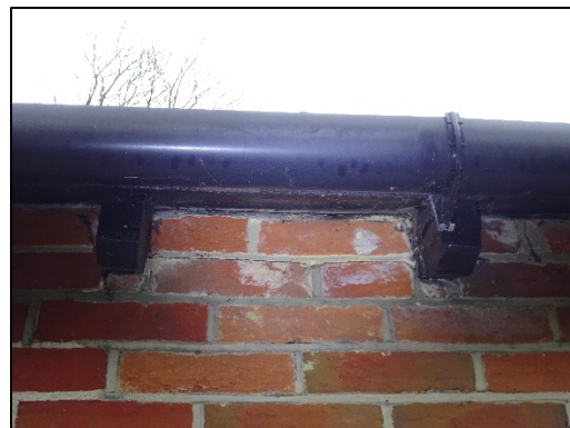
Figure 2 – eaves with internal beams visible on the southern elevation of the pitched extension
