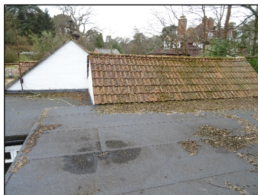
Figure 5 – flat roof meeting the northern roof face of the pitched extension and the northern gable end of the main section of the house
