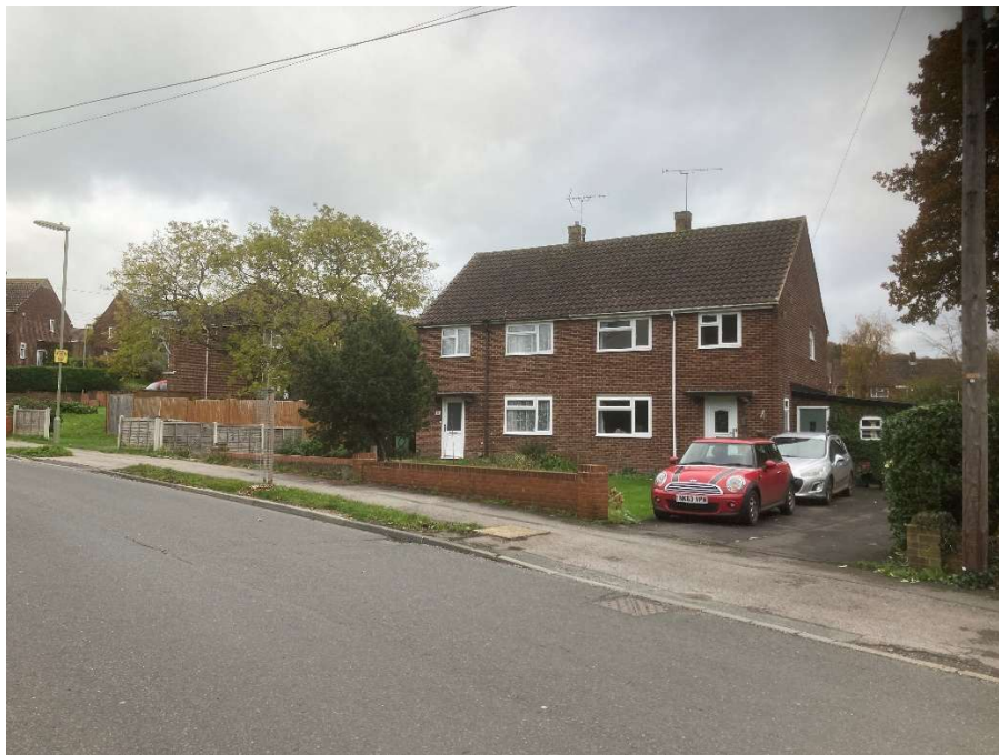
Fig. 2 – Photo of 6-8 Sedgwick Road with the parking area and side area of no. 6 shown on the right.
