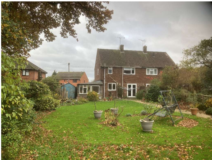
Fig. 6 – Photo showing the rear elevation of 6-8 Sedgwick Road (no.6 on left).
