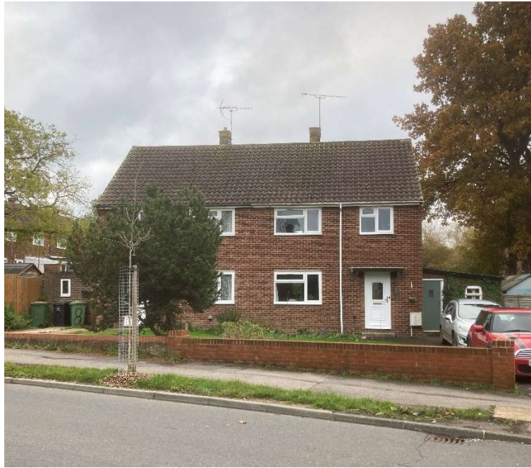
Fig.1 – Photo of the front elevations of 6-8 Sedgwick Road (no.6 on right).
