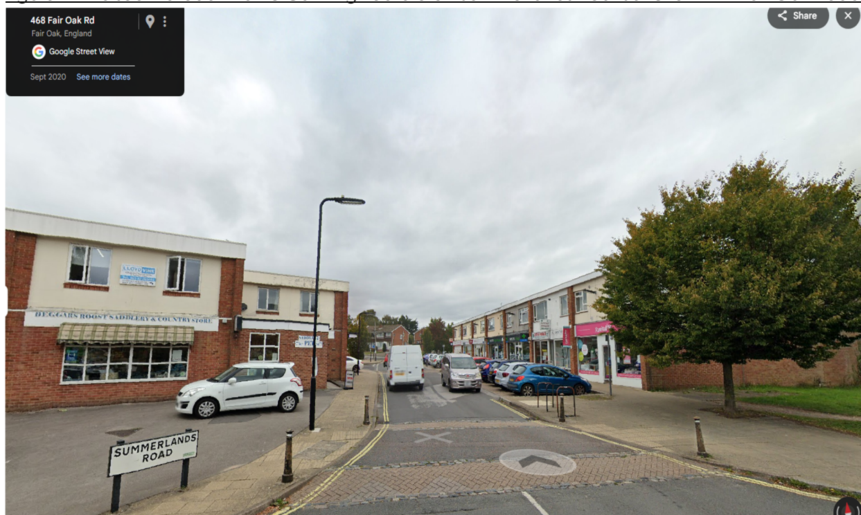
Figure 1 – Raised Plateaux Traffic Calming Feature on Summerlands near Junction with Fair Oak Road
