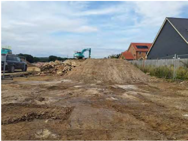
Description Reduced dig Area D
