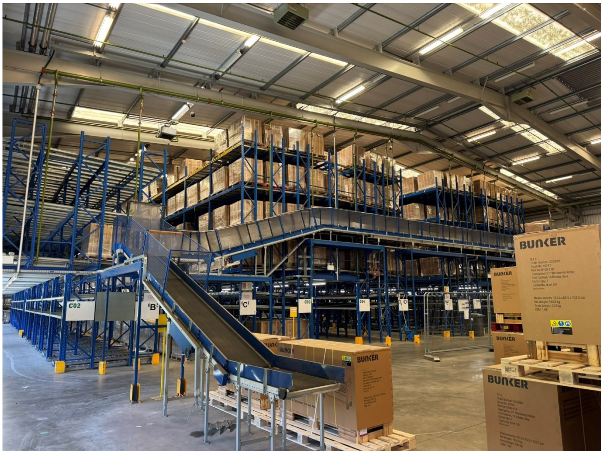
Internal view of the building with the racking and conveyors, which are being removed.
