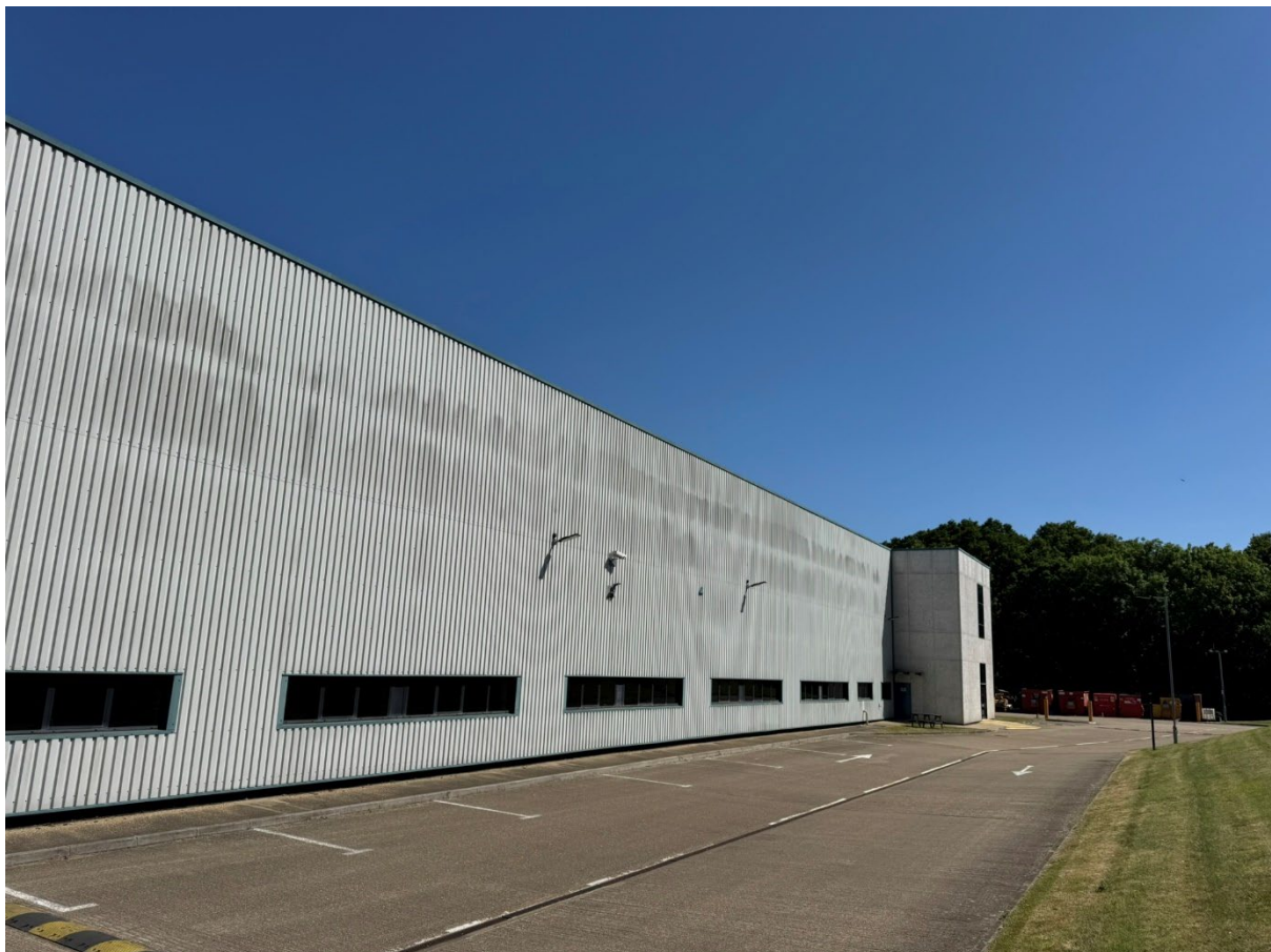
West elevation of existing building with existing entrance at the right hand end of the image.
