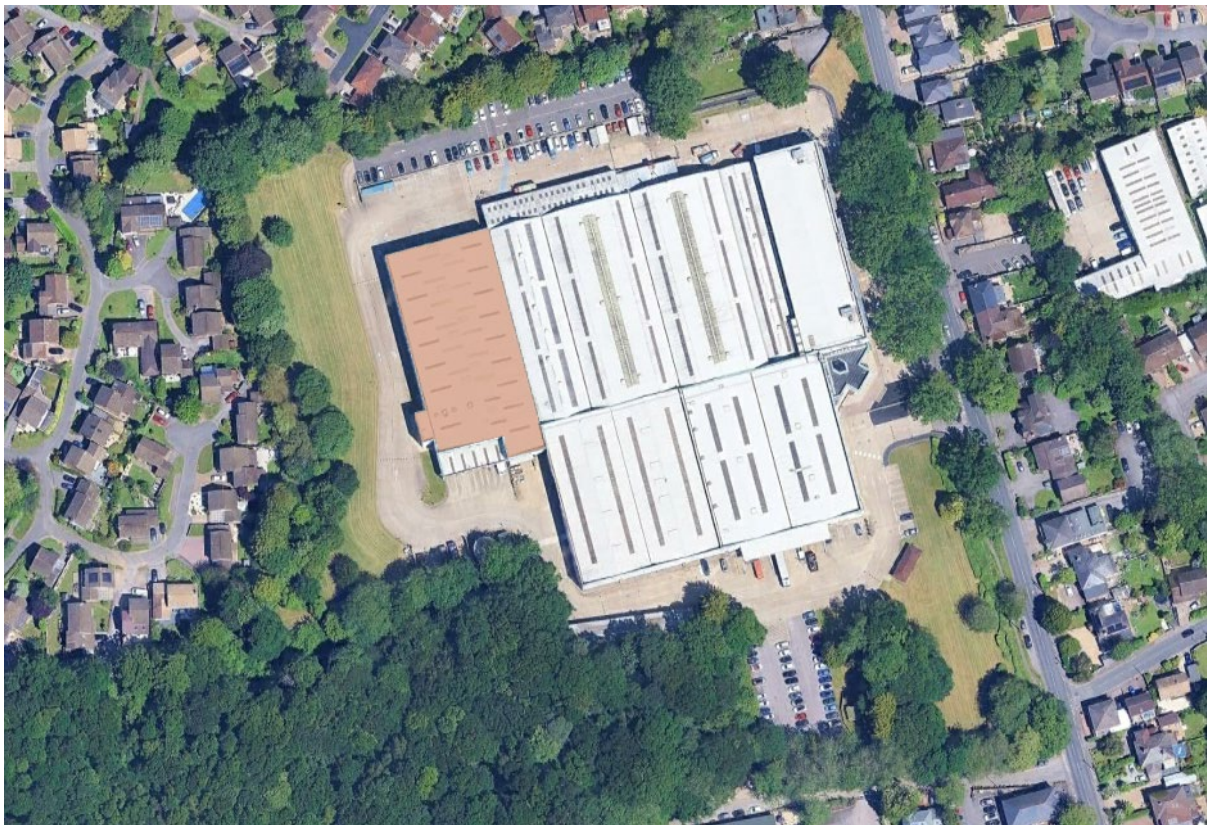
Aerial photograph showing building subject to this change of use application hatched pink.
